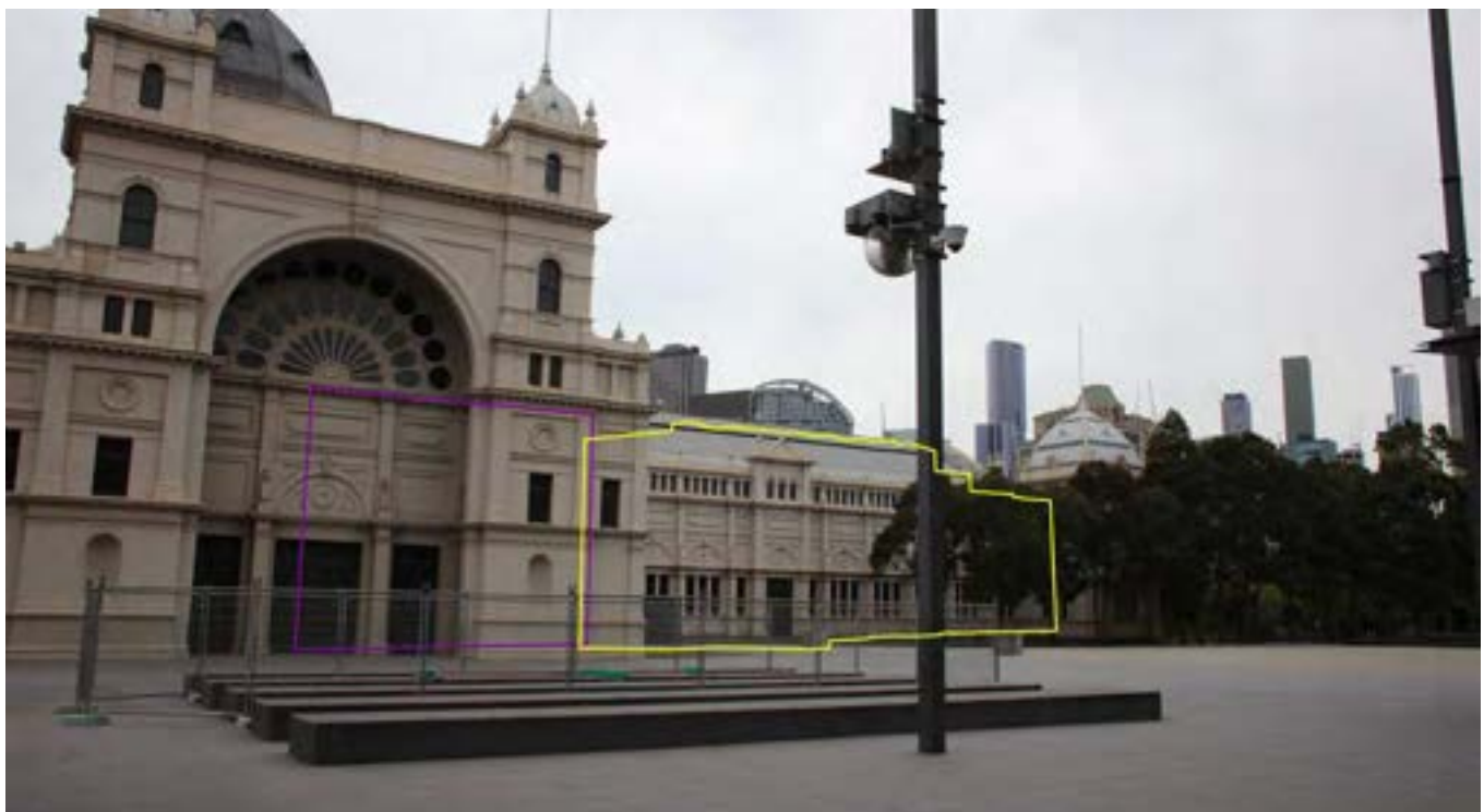
Testing of proposed 'concealment height' of built form (outline). Note: the proposed development is fully concealed this camera location
