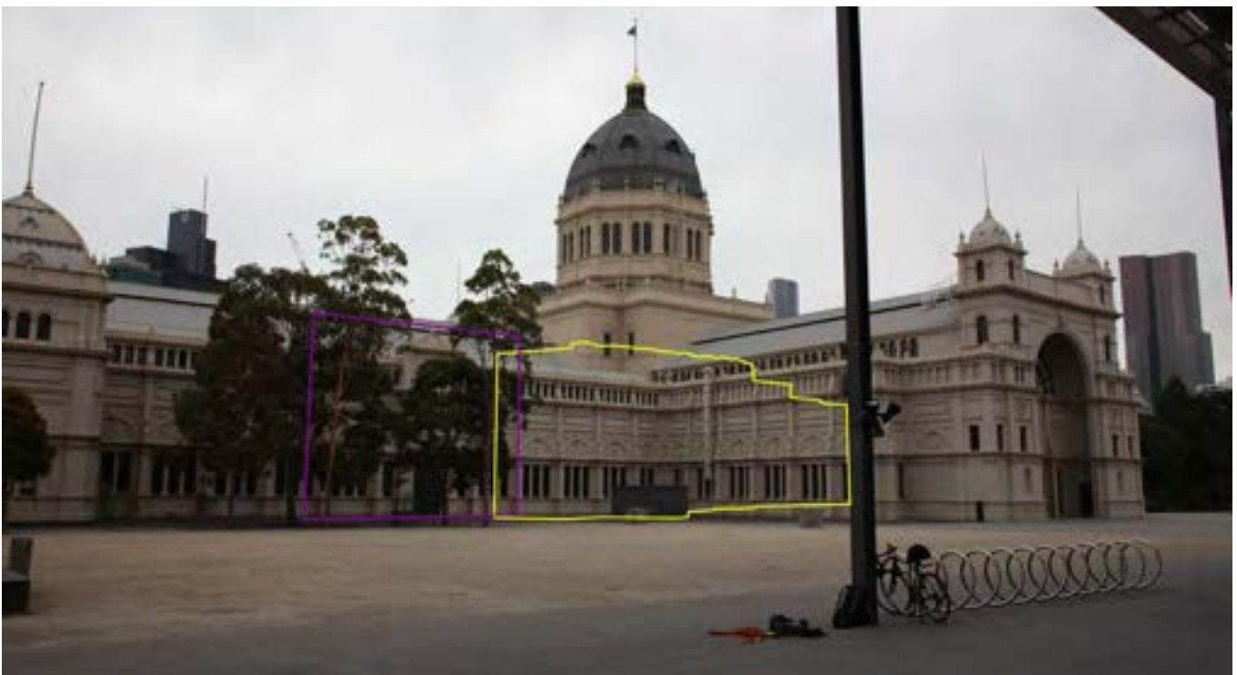
Testing of proposed 'concealment height' of built form (outline). Note: the proposed development is fully concealed this camera location
