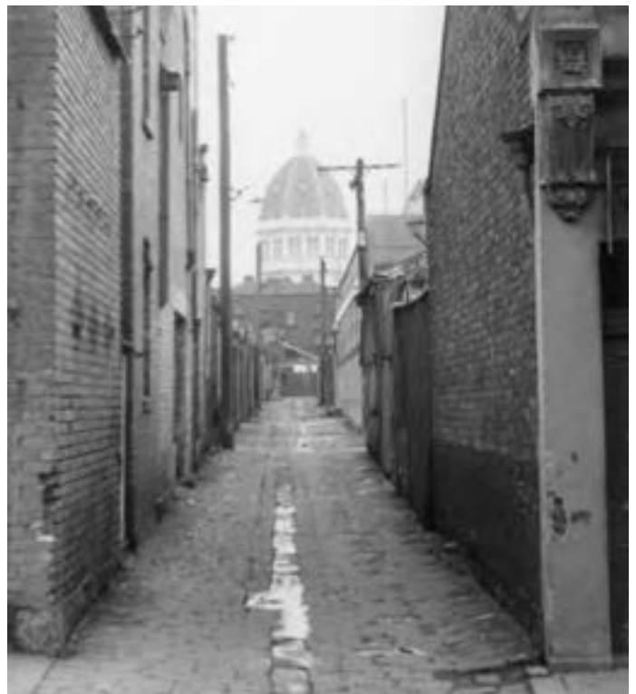
Looking west along a laneway between Gertrude & Marion Streets ca1958 (University of Melbourne Archives Reference: 1965.0004.00022).
