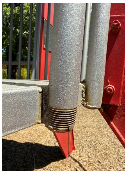
2025, Benalla Playground Rocket, galvanised pipe construction detail.
