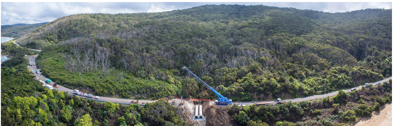
Replacing culverts near Wye River. (Image: Department of Transport)
