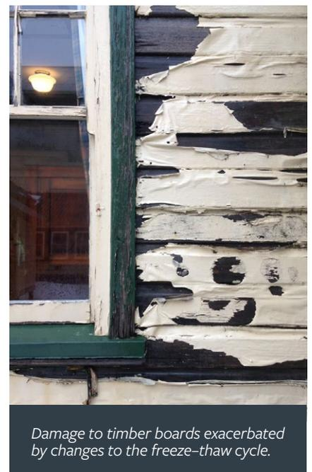
Damage to timber boards exacerbated by changes to the freeze-thaw cycle.
