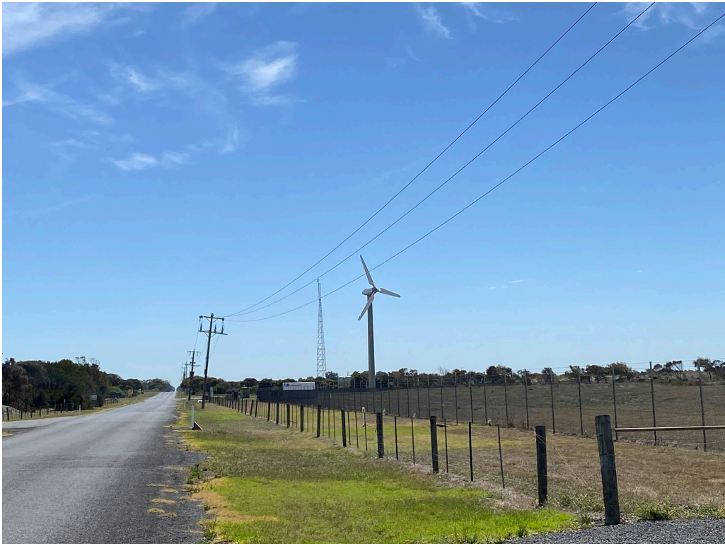
2025, the Demonstration Wind Turbine viewed from Blackrock Road, to the south of the turbine, Source: Heritage Victoria
