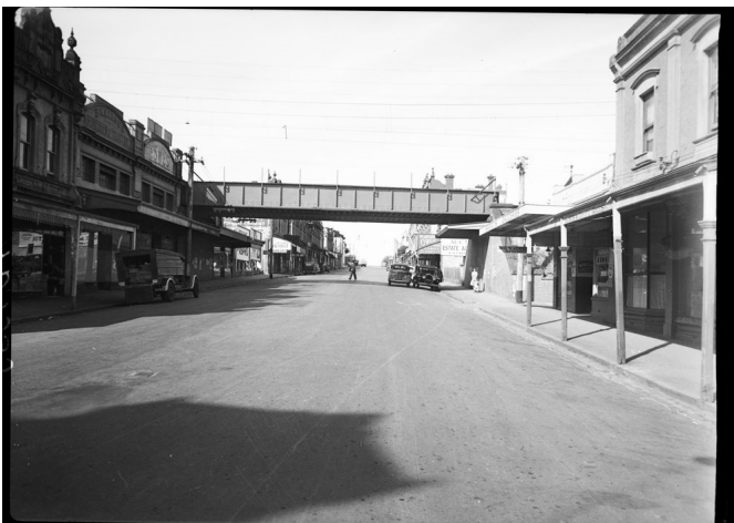
Undated (c1930), Railway bridge over Auburn Road, Source: PROV VPRS 12800/P0003, ADV 1365.
