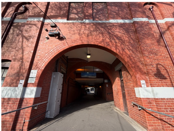
Transverse passageway from north elevation of downside station building below railway line, Source: Heritage Victoria.
