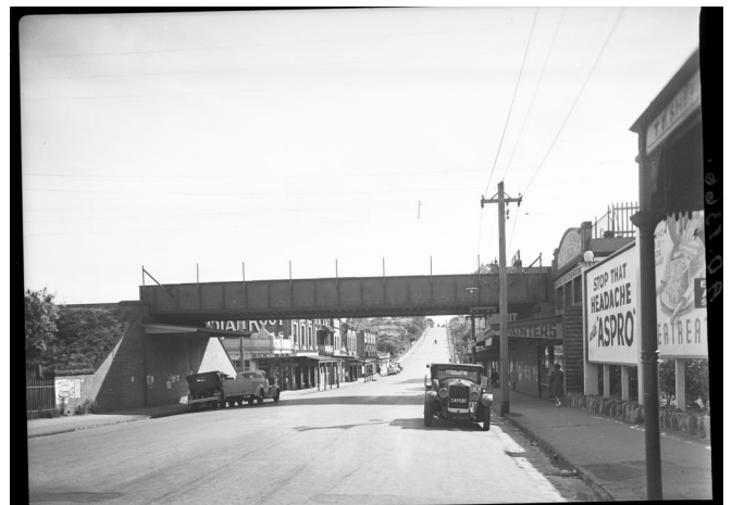
Undated (c1930), Railway bridge over Auburn Road, Source: PROV VPRS 12800/P0003, ADV 1366.
