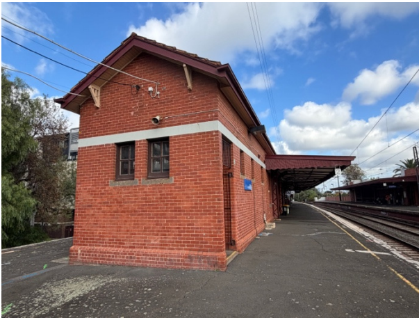
Island platform station building, Source: Heritage Victoria
