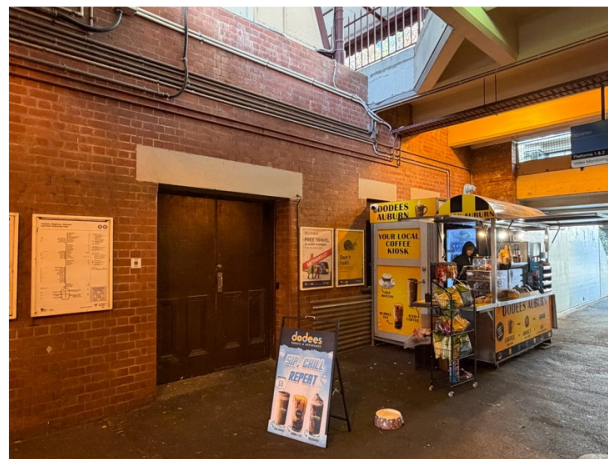
Former booking office/station master's office within transverse passageway. Lightwell from island platform above, Source: Heritage Victoria.
