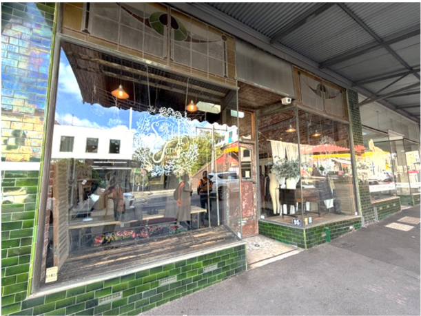
Shopfronts to north of rail bridge, Source: Heritage Victoria.
