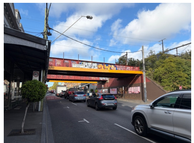
Rivetted steel railway bridge (original bridge in foreground, 1963 bridge to south), Source: Heritage Victoria.
