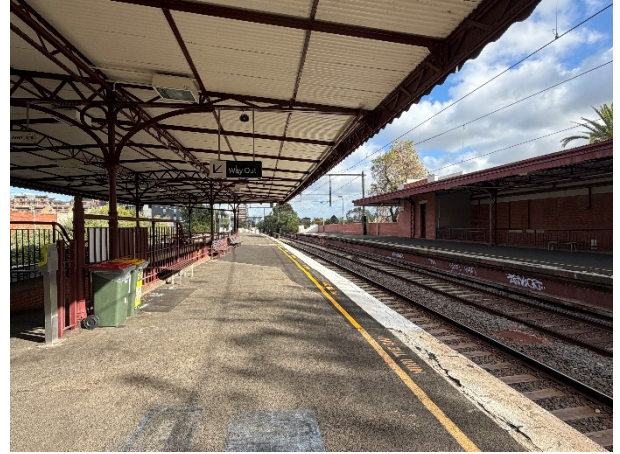
Island platform with broad canopy with open web trusses and decorative wrought iron brackets, Source: Heritage Victoria
