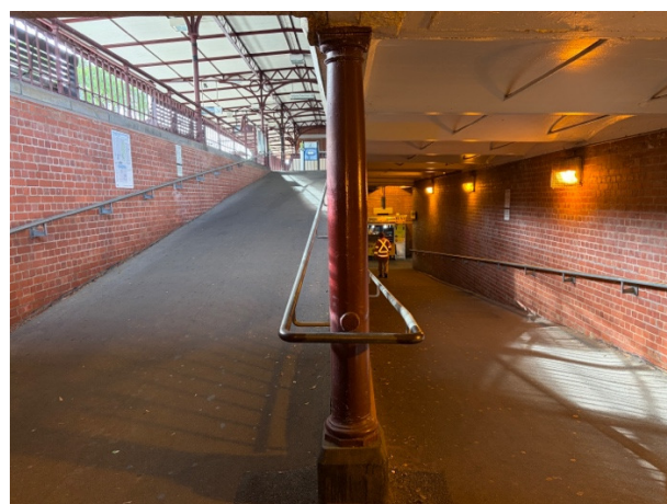
Pedestrian ramp from transverse passageway to island platform, Source: Heritage Victoria.
