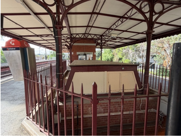
Island platform with station building, broad canopy and clerestory form skylight, Source: Heritage Victoria.
