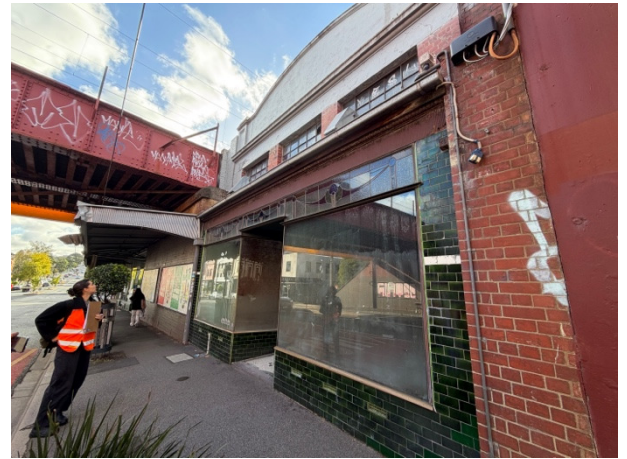
Shopfront between rail bridges, Source: Heritage Victoria.
