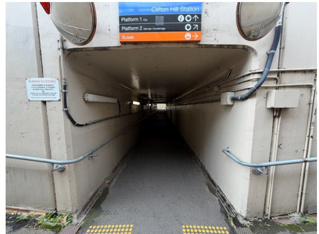
2026, Entrance to pedestrian underpass from west (Hoddle Street), Source: Heritage Victoria.
