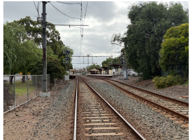
2026, Railway corridor looking north from Ramsden Street, Source: Heritage Victoria.
