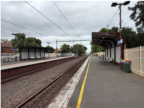
2026, Railway corridor looking south to Ramsden Street with later shelters, Source: Heritage Victoria.
