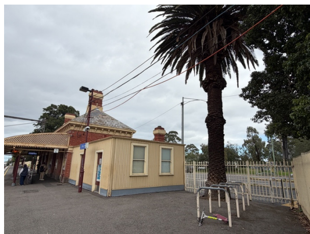
2026, Downside station building, former Porters Store and mature Canary Island Palm (Phoenix canariensis), Source: Heritage Victoria.
