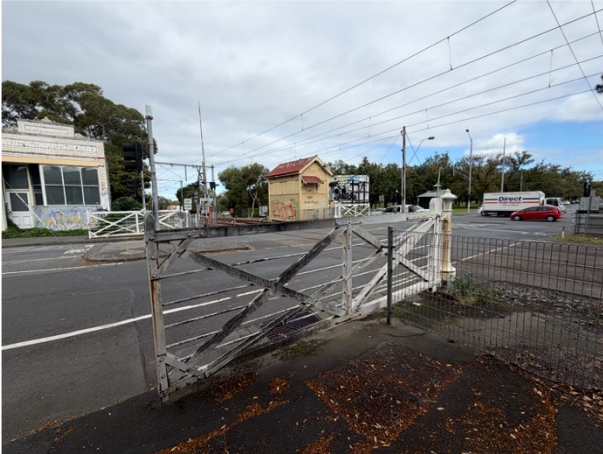
2026, Timber railway gates mounted on cast-iron piers at Ramsden Street level crossing, Source: Heritage Victoria.
