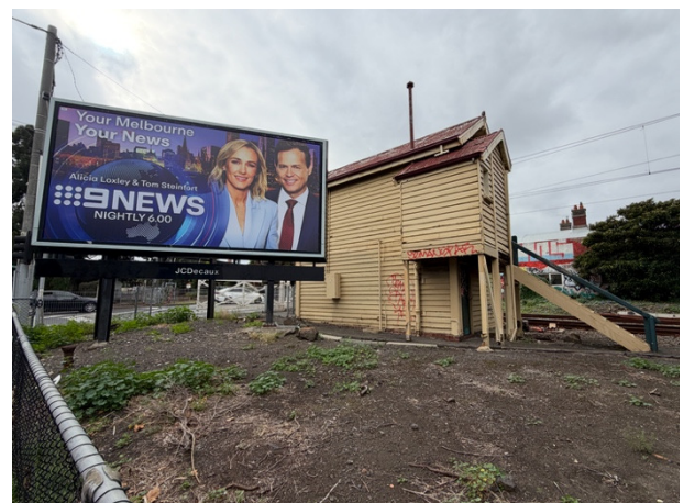
2026, Signal Box A and timber stairs to the south, Source: Heritage Victoria.
