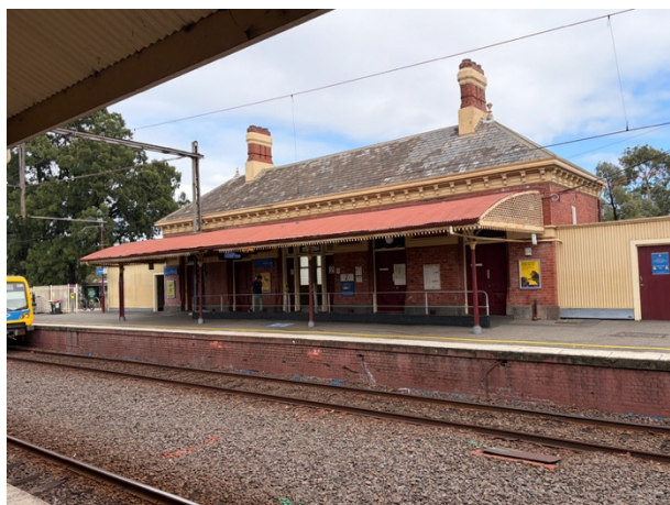
2026, Clifton Hill downside station building east (platform) elevation, Source: Heritage Victoria.
