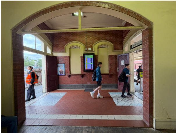
2026, Downsides station building foyer and covered ticket windows, Source: Heritage Victoria.
