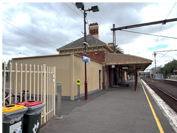
2026, Downside station building and corrugated metal-clad former men's bathrooms to south, Source: Heritage Victoria.
