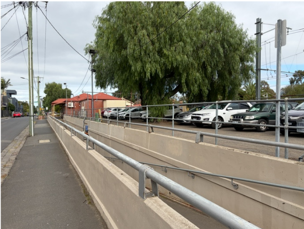
2026, Ramp to pedestrian underpass and at-grade car park north of upside station building, Source: Heritage Victoria.
