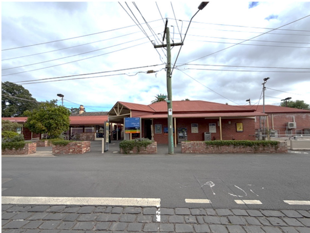
2026, Upside station building east (John Street) elevation, Source: Heritage Victoria.
