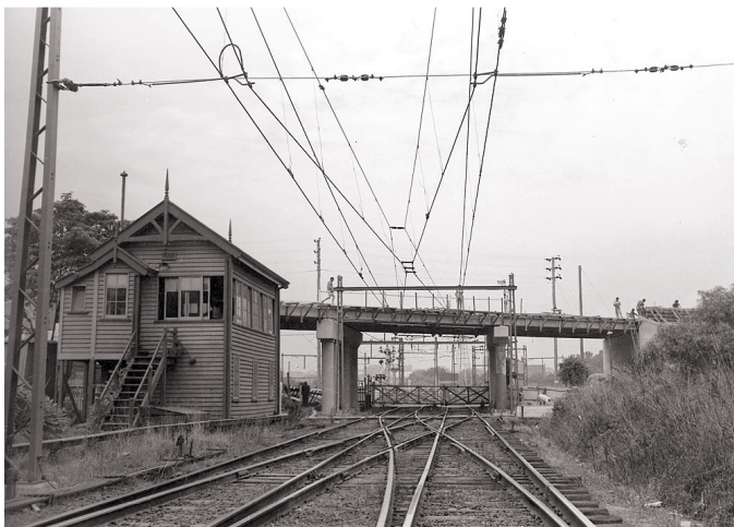
1957, Clifton Hill B Signal Box during construction of the Heidelberg Road overpass, Source: Victorian Railways https://www.victorianrailways.net/photogallery/suburb/gal04/chillbbox.html
