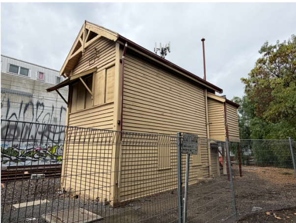
2026, Signal Box B near Heidelberg Road overpass further north and west of railway corridor, Source: Heritage Victoria.
