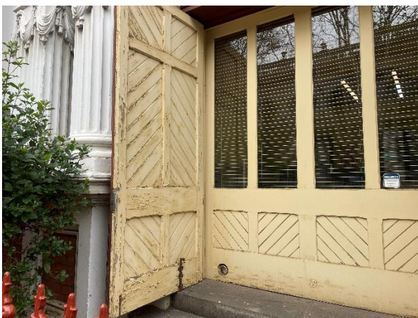
2026, Main entrance with later glazed timber infill panels and original doors with diagonal panelling, Source: Heritage Victoria.
