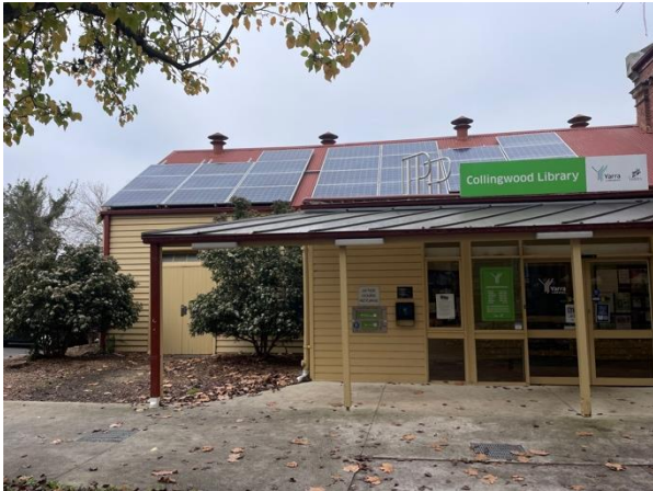
2026, Former hall with later entrance addition, Source: Heritage Victoria.
