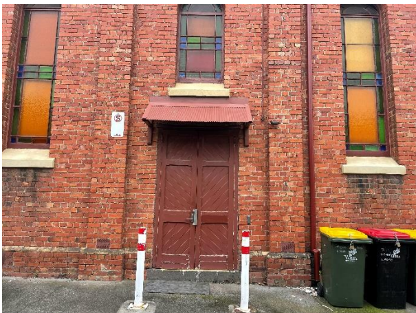
2026, Southern opening to west elevation, Source: Heritage Victoria.
