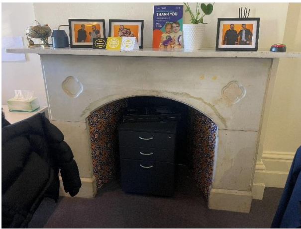
2026, Stone fireplace with quatrefoil carvings and tiled firebox in former Drawing Room at first floor, Source: Heritage Victoria.
