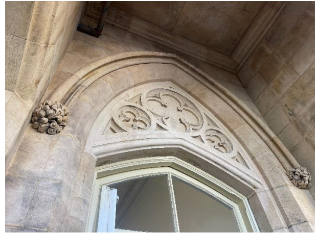
2026, Quatrefoil and trefoil plate tracery above the main entrance door, Source: Heritage Victoria.
