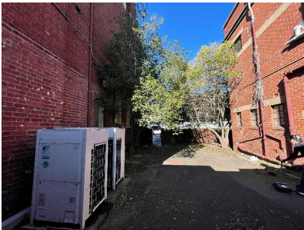
2026, Courtyard to the west of the bank (left), Source: Heritage Victoria.
