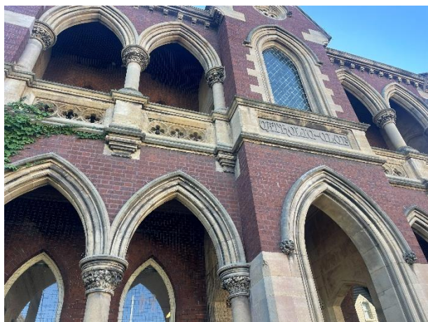
2026, Detail of the principal (south) elevation, Source: Heritage Victoria.
