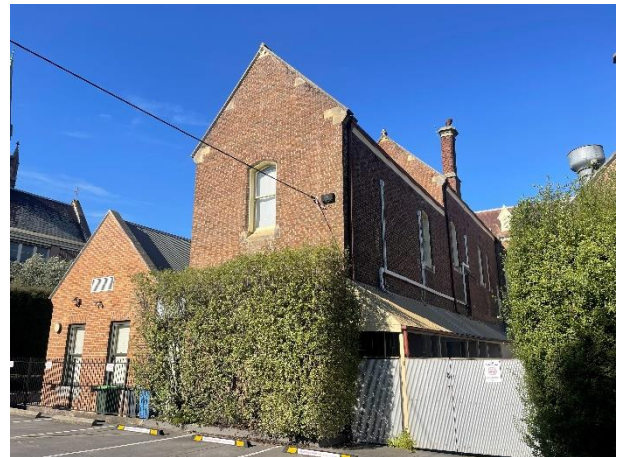
2026, Later addition (left) and rear wing of the bank (right), Source: Heritage Victoria.
