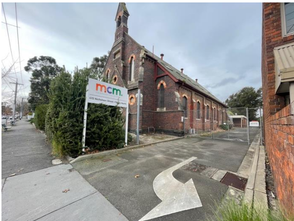
2026, South elevation with laneway (right) along the southern boundary of the site, Source: Heritage Victoria.
