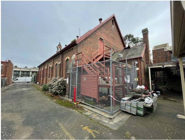
2026, East elevation with fire stair, Source: Heritage Victoria.
