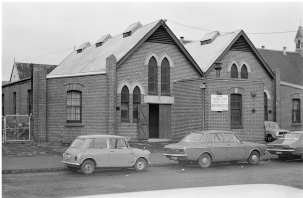
c1970-74, Methodist Sunday School/Hall (demolished in the 1970s) fronting Church Street, northeast of the Methodist Church (behind at right), Source: State Library Victoria, ID 9939658317607636.
