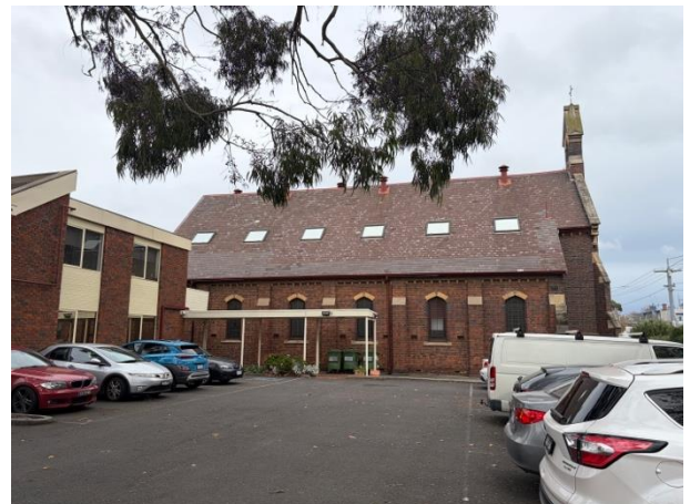
2026, North elevation with residential facility to left, Source: Heritage Victoria.
