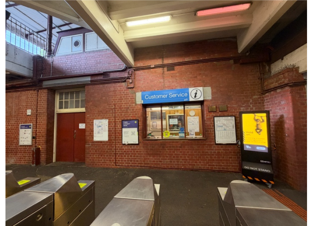
2026, Customer service office and lightwell within transverse passageway, Source: Heritage Victoria.
