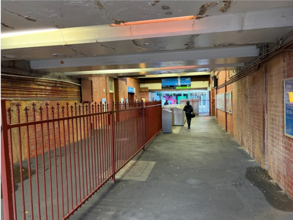
2026, Transverse passageway below railway line, looking south, Source: Heritage Victoria.
