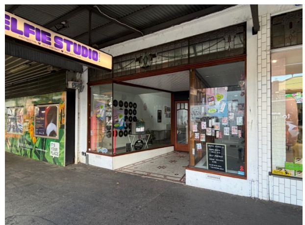
2026, Shopfront between two rail bridges, Source: Heritage Victoria.
