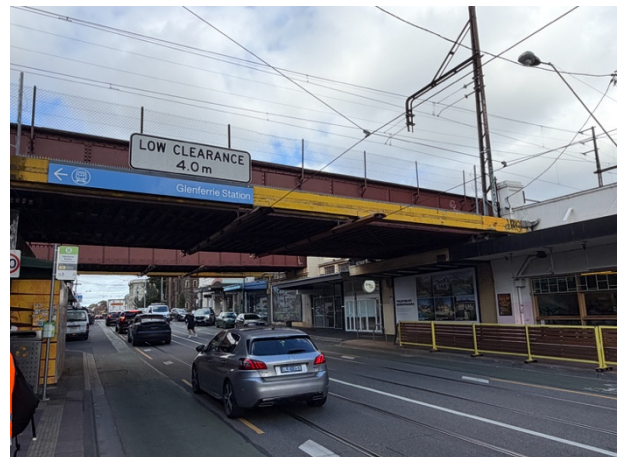
2026, Rivetted steel railway bridge over Glenferrie Road and 1963 bridge to south (behind), Source: Heritage Victoria.
