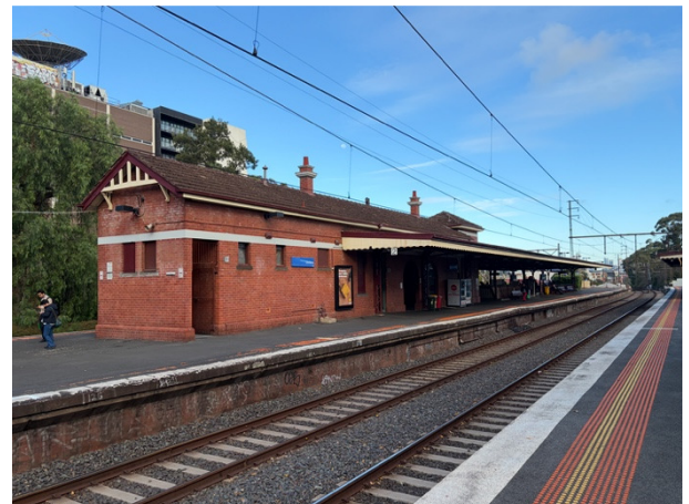
2026, Island platform station building, Source: Heritage Victoria.
