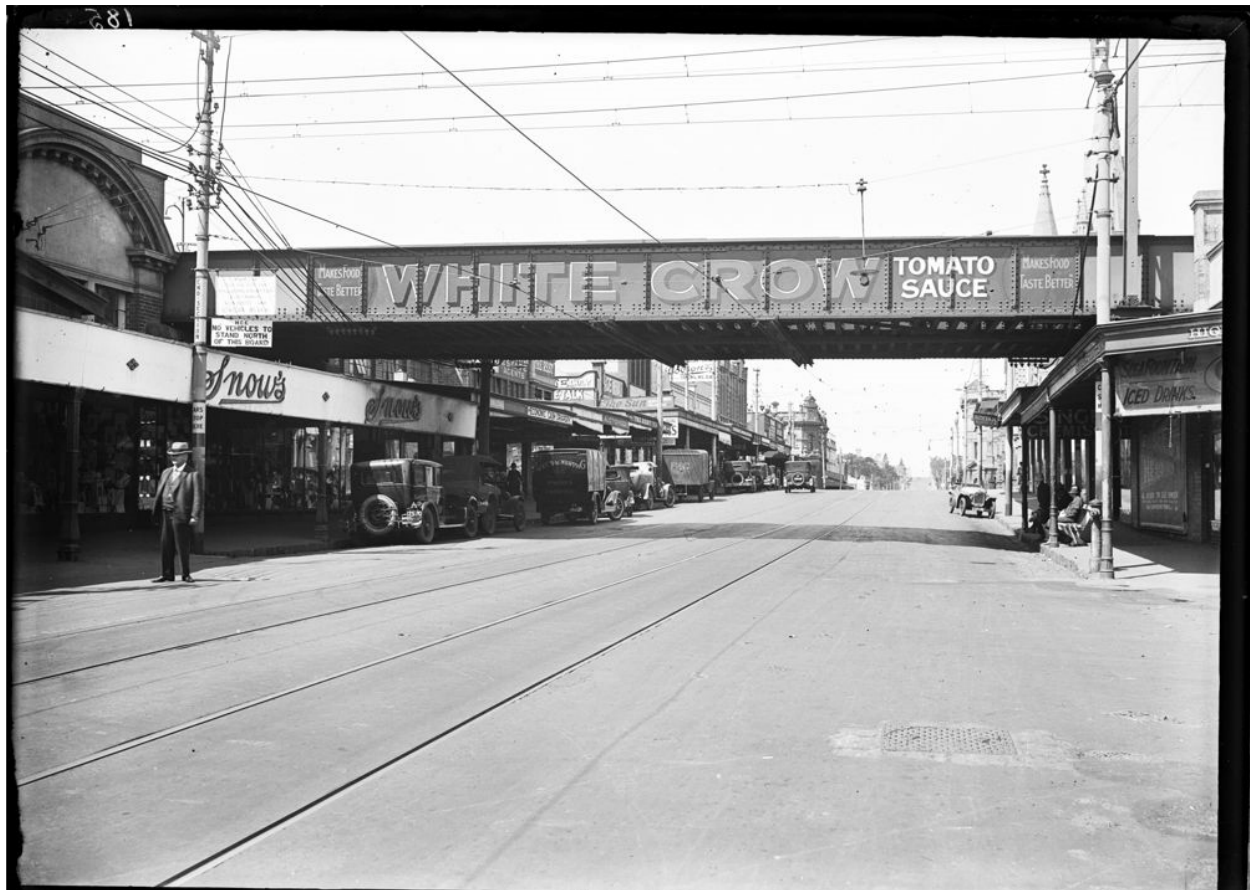
Undated (c1930), Railway bridge over Glenferrie Road: PROV VPRS 12800/P0003, ADV 0185.
