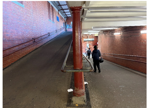
2026, Pedestrian ramp from transverse passageway to downside platform, Source: Heritage Victoria.
