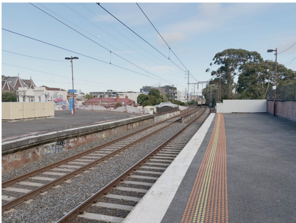
2026, Downside platform (right) and island platform (left), rivetted steel railway bridge (centre) over Glenferrie Road, Source: Heritage Victoria.
