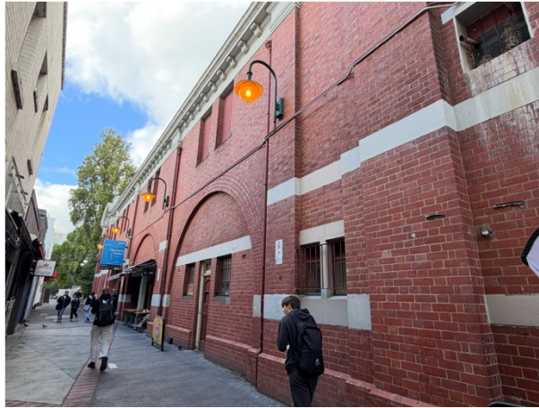
2026, North elevation of Glenferrie Station downside station building looking east from Don Arcade, Source: Heritage Victoria.
