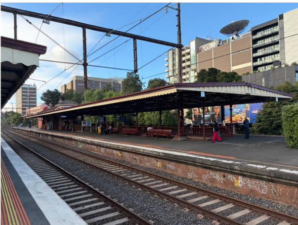
2026, Island platform with broad canopy above pedestrian ramp, Source: Heritage Victoria.
