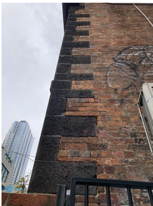
2026, Bluestone quoins on northside of building, Source: Heritage Victoria.
