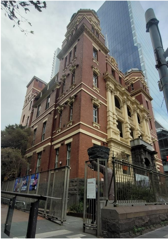
June 2026. Former Queen Victoria Hospital Pavilion from Lonsdale Street, facing north-east (Source: Heritage Victoria).
