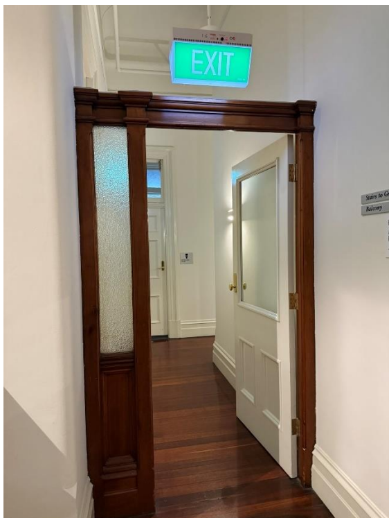
June 2026. Timber door frame with glazing (Source: Heritage Victoria).
