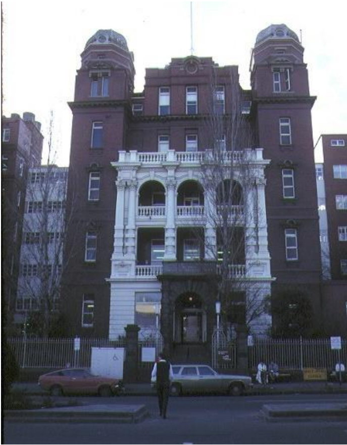
July 1984. 'Block E', the main entry and administration block, with wards on the upper floors. Note the corridors connecting to the adjacent pavilions at the rear (Source: Heritage Victoria file photograph).
