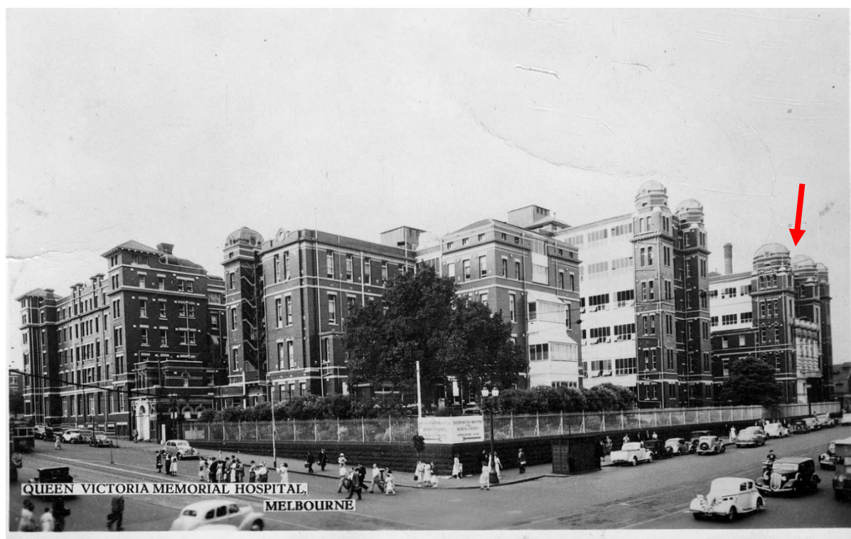
c. 1940s. Queen Victoria Memorial Hospital, corner of Swanston and Lonsdale Streets. Note the perimeter fence. Balconies have had glazing added. Extant pavilion marked with an arrow. (Source: State Library of Victoria).
