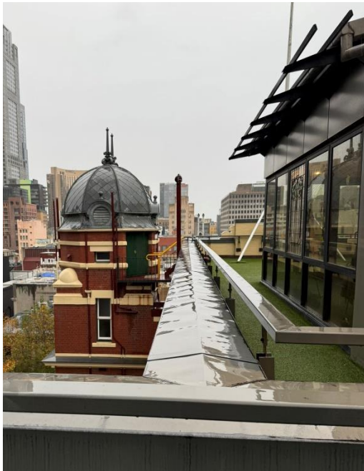
June 2026. Facing south towards the eastern tower and cupola, new roof function space at right (Source: Heritage Victoria).
