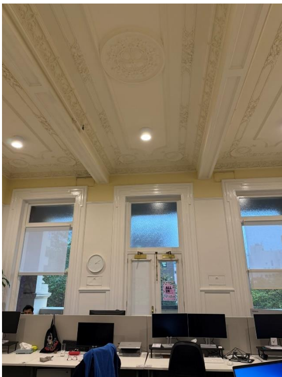
June 2026. First floor, former boardroom with highly decorative ceiling (Source: Heritage Victoria).
