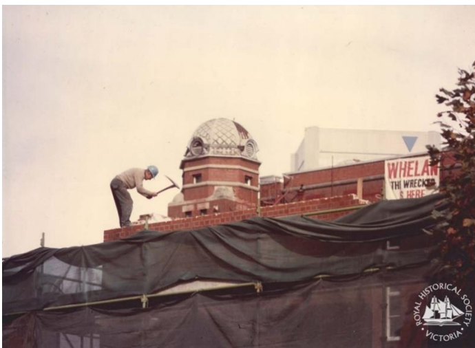
1990. Demolition of the Queen Victoria Hospital, Lonsdale Street, Melbourne (Photo: Kevin Patterson. Source: Royal Historical Society of Victoria).
