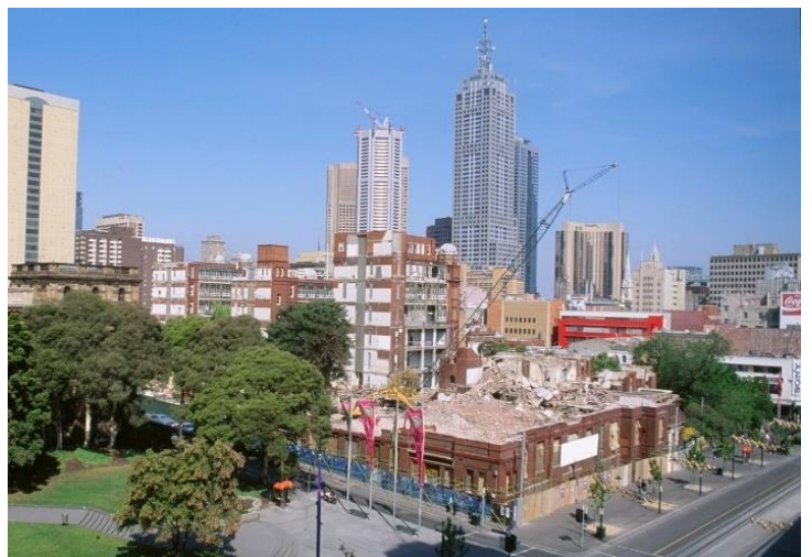
1993. Queen Victoria Hospital from Jensen House, taken during demolition (Photo: Adrian Flint. Source: State Library of Victoria).
