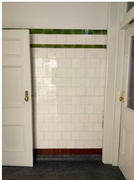
June 2026. Original hospital wall tiles on the second floor (Source: Heritage Victoria).
