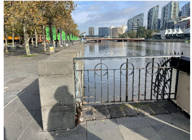
2026, Later fixed metal fence and decorative cast iron fan to west balustrade end (right), Source: Heritage Victoria.
