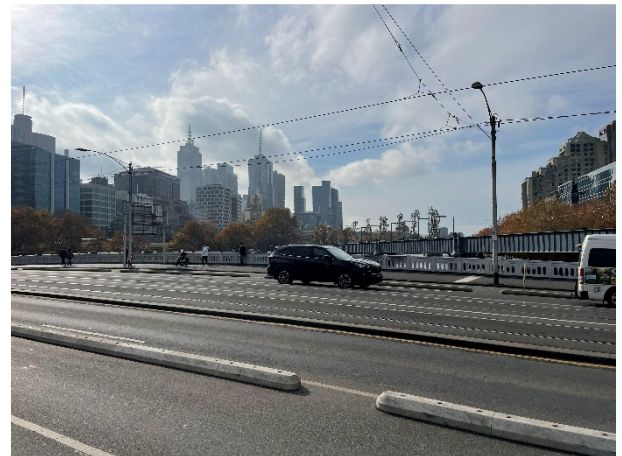
2026, Carriageway to Queens Bridge with asphalt surface and traffic infrastructure (looking east), Source: Heritage Victoria.
