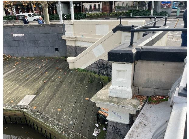
2026, Northwestern bluestone abutment and staircase leading to timber decked landing, Source: Heritage Victoria.
