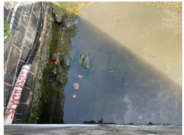
2026, Remnant basalt likely from earlier Falls Bridge, southeast of Queens Bridge, Source: Heritage Victoria..
