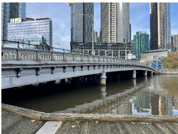
2026, West side of Queens Bridge and timber decked landing (foreground) looking south, Source: Heritage Victoria.
