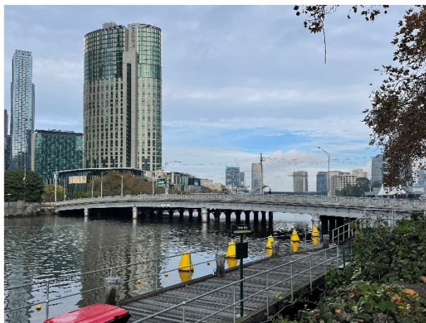
2026, Queens Bridge east view from north of riverbank, Source: Heritage Victoria.
