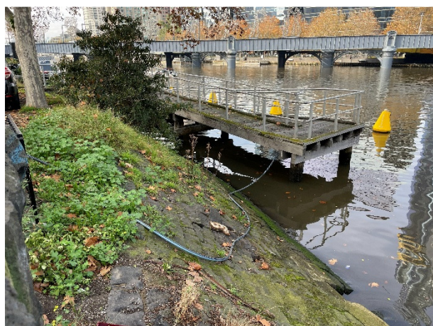
2026, Bluestone embankment northeast of Queens Bridge, Source: Heritage Victoria.
