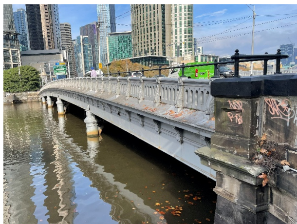
2026, East side of Queens Bridge and north abutment (right) looking south, Source: Heritage Victoria.
