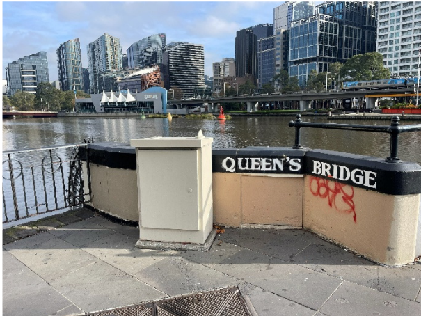
2026, Southwestern end of Queens Bridge with cast-iron handrail, Source: Heritage Victoria.
