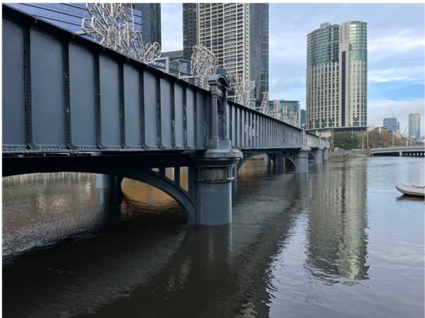
2026, Western side of bridge, Source: Heritage Victoria.
