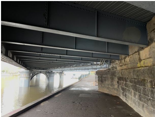
2026, Underside of eastern carriageway (above) and north bank abutment (right), Source: Heritage Victoria.
