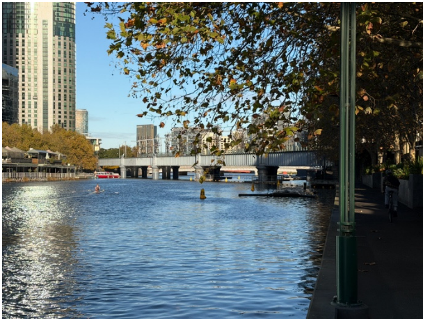
2026, Sandridge Railway Line Bridge east view, from north of riverbank, Source: Heritage Victoria.
