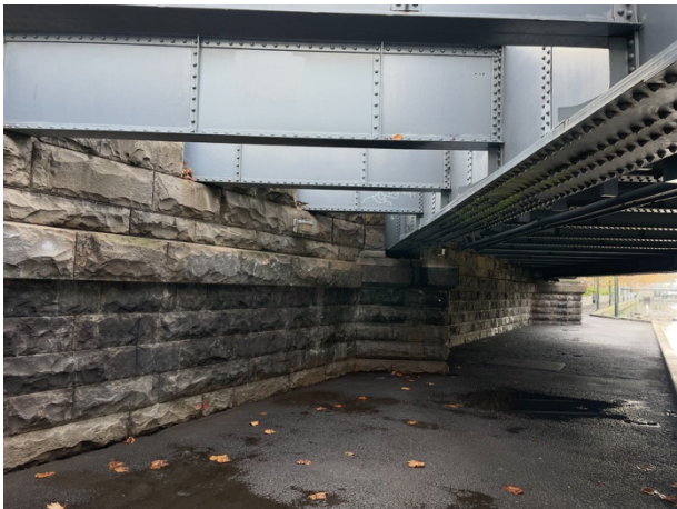
2026, North bank bluestone abutment, Source: Heritage Victoria.
