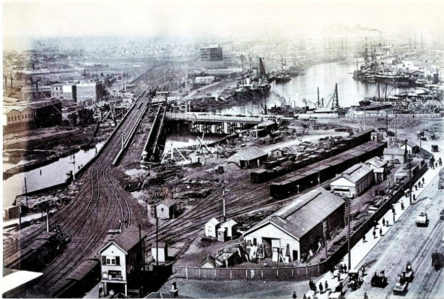
Melbourne; Yarra River with old wooden bridge and Sandridge Railway Bridge under construction.
