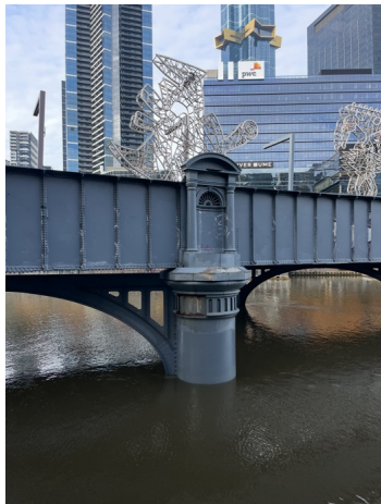
2026, Pier detail with artwork above, Source: Heritage Victoria.
