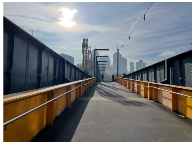
2026, Ramp from Southbank to the bridge shared user path (looking north), Source: Heritage Victoria.
