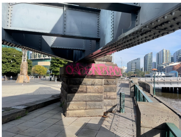
2026, Bluestone abutment on south bank supporting steel girders at southwest corner, Source: Heritage Victoria.
