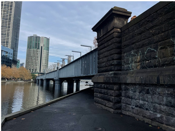
2026, North bank bluestone abutment and eastern side of bridge, Source: Heritage Victoria.
