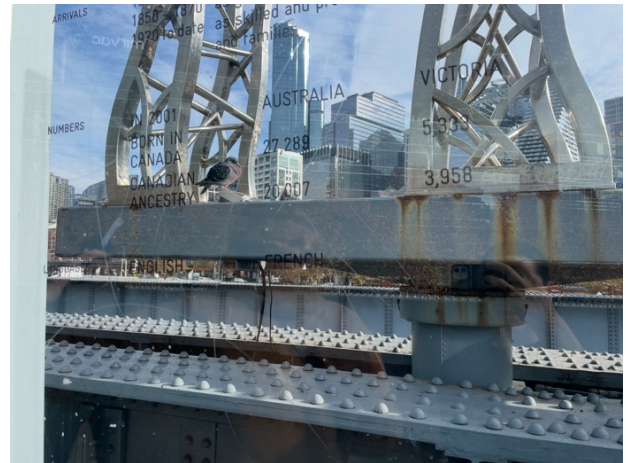
2026, Parallel steel girders with detail of etched glazing with immigration details in foreground, Source: Heritage Victoria.
