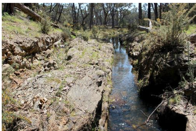
Figure 5. Stone-cut tail race in Three Mile Creek adjacent to sludge dam (Peter Davies 2024)
