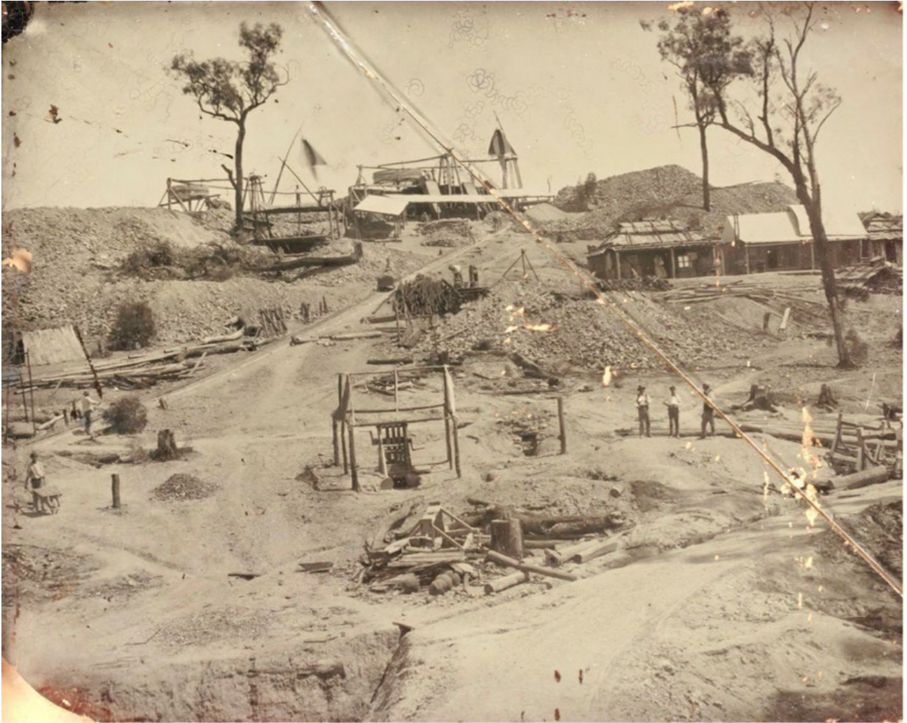
Figure 16. Balaclava Hill from the north c.1859 with workings on the summit including wind sails for shaft ventilation and a horse whim for raising ore (State Library Victoria)
