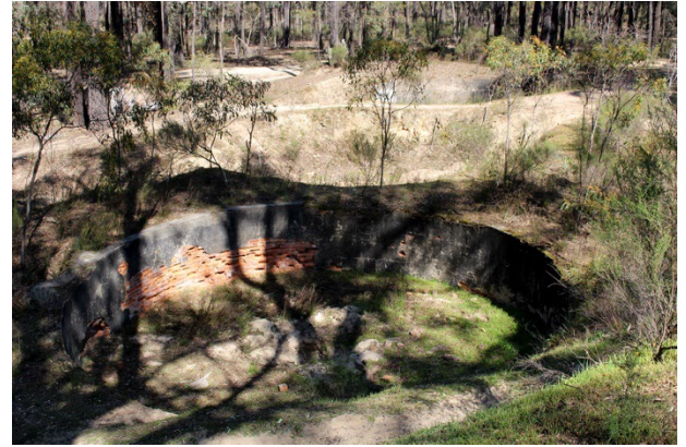
Figure 8. Three cyanide vats used to reprocess quartz tailings from the Balaclava Hill Mine c.1900 (Peter Davies, 18 September 2024)
