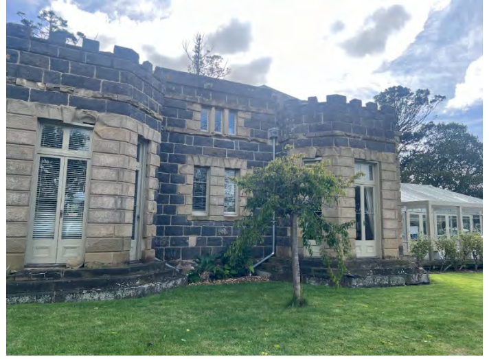
2025. Barwon Bank southern elevation. Source: HV.
