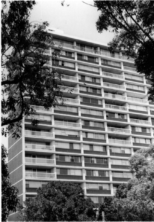
c. 1967-75, north elevation, photographed by John T Collins, Source: State Library of Victoria.
