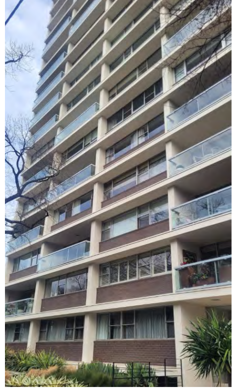
2026, arrangement of balconies, windows and spandrels to the north elevation, Source: Heritage Victoria.
