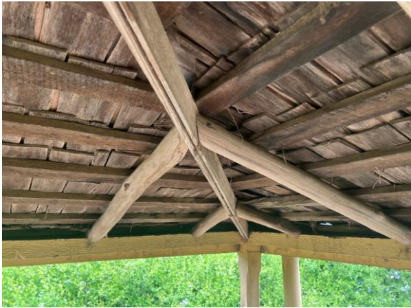
2025. Timber shingles visible under verandah roof.
