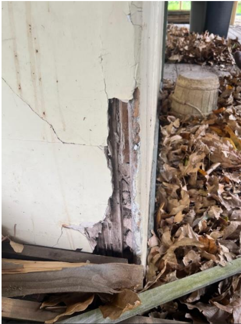
2025. Failing daub to exterior wall.
