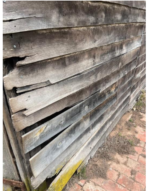
2025. Weathered timber members to exterior wall of shed.
