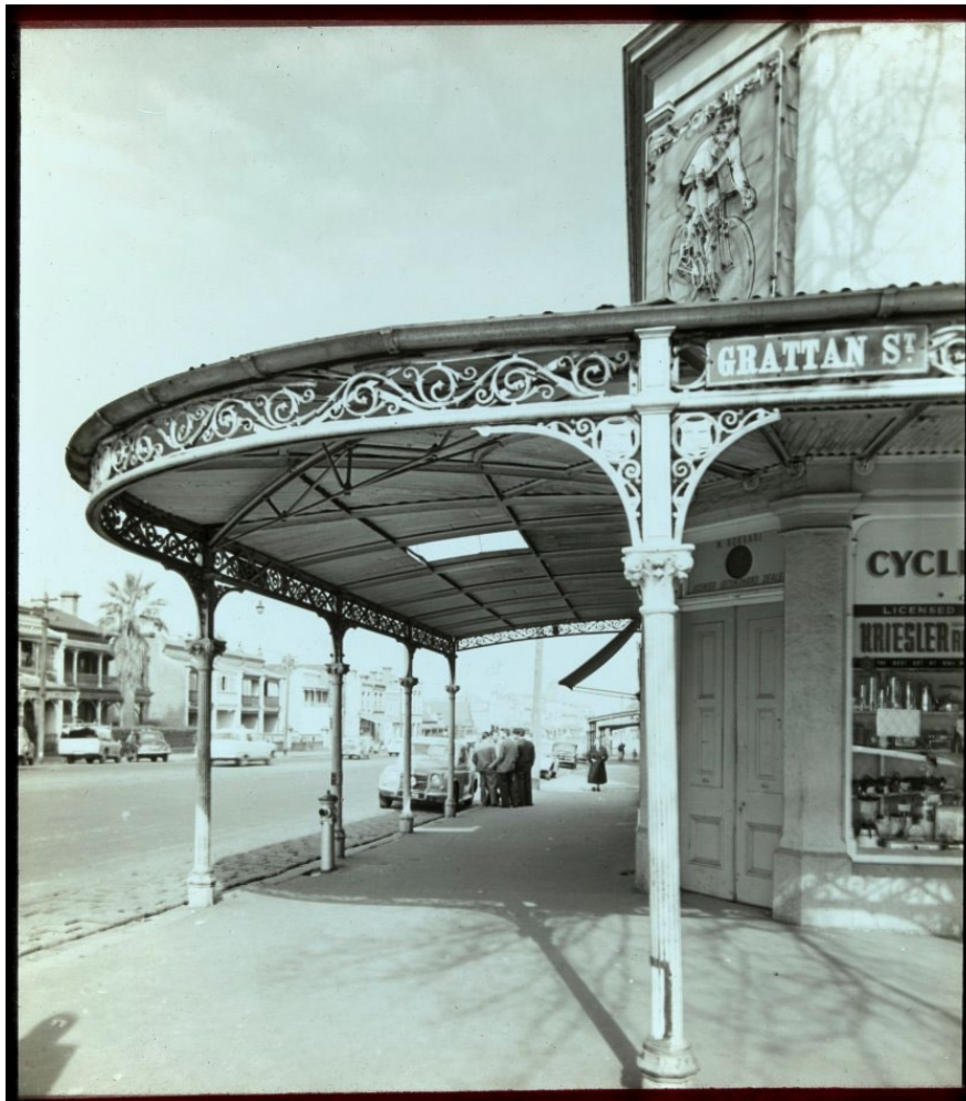
1950-60, Borsari's Corner with signage in place, Source: State Library of Victoria.
