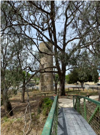
2025, Wunghnu Water Tower as viewed from the bridge over Nine Mile Creek. This image indicates the proximity of the tower to the Creek. Source: Heritage Victoria.
