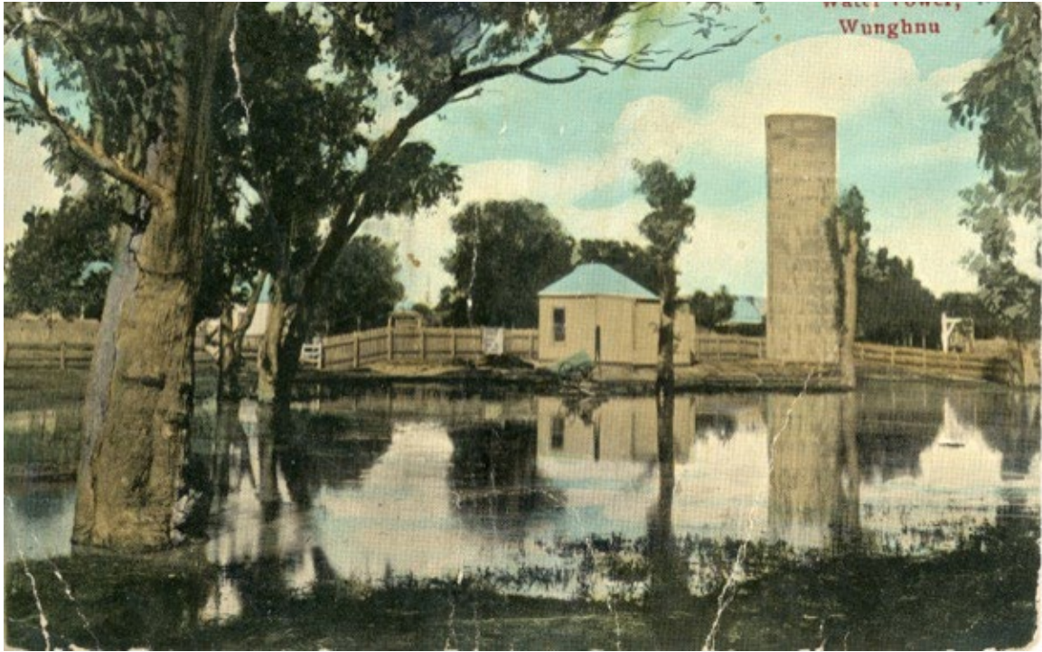
1909, Water Tower at Wunghnu, Postcard (hand painted), standpipe Water Tower with pumping/engine house (to the left), ground level structure (to the right) likely used to fill up a portable tank or barrel on the back of a cart. Source: Lost Shepparton Facebook page .
