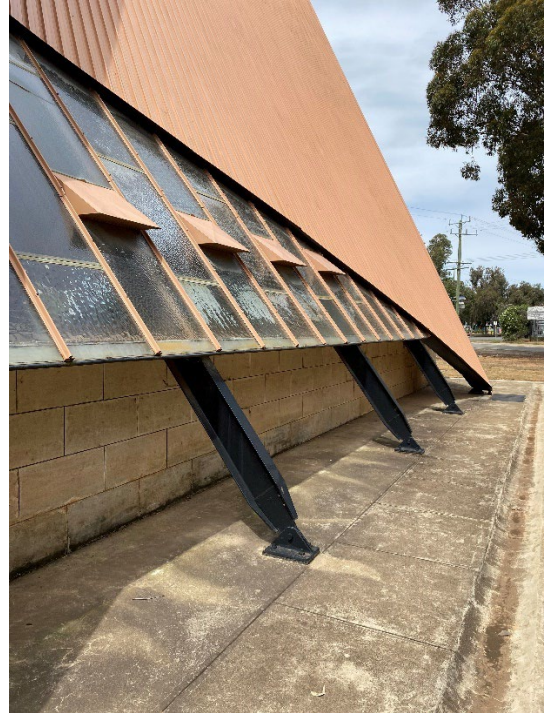
2025, detail of structural A-frame, with limestone walls visible behind. Source: Heritage Victoria.
