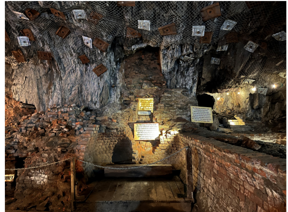
Figure 16. Brick lined flue and ventilation shaft (Peter Davies)
