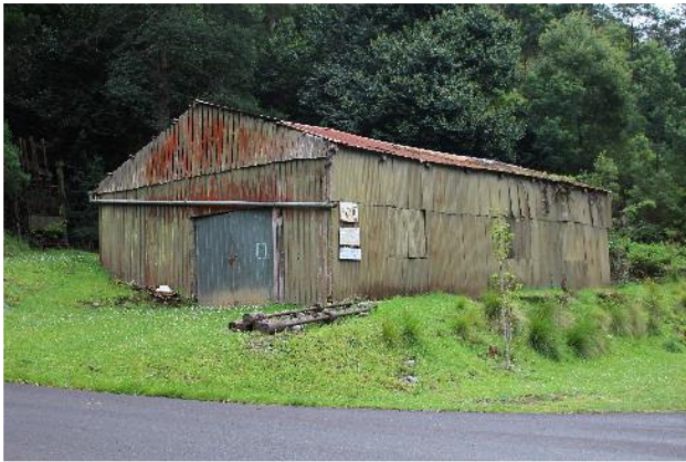
Figure 5. Paling and corrugated iron shed from 1980s on site of Long Tunnel Extended stamp battery (Peter Davies)
