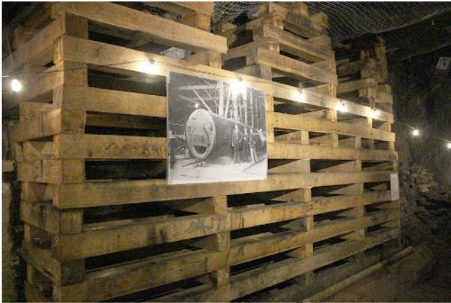
Figure 15. Timber sets or cribs in machinery chamber of Long Tunnel Extended gold mine (Peter Davies)
