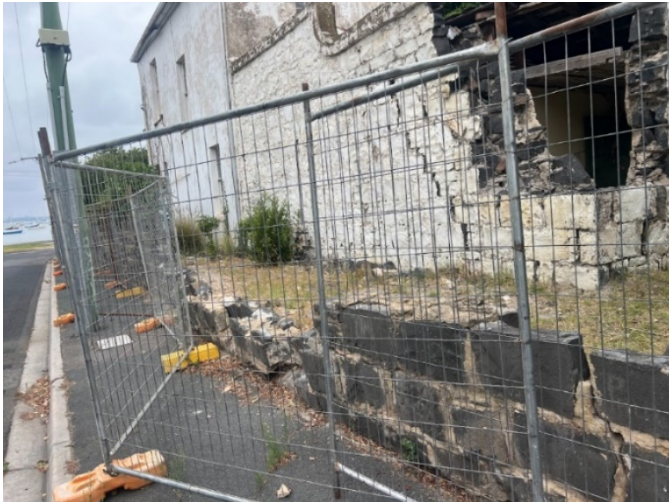
2026. Dismantled section of bluestone wall and dismantled skillion-roofed service wing.
