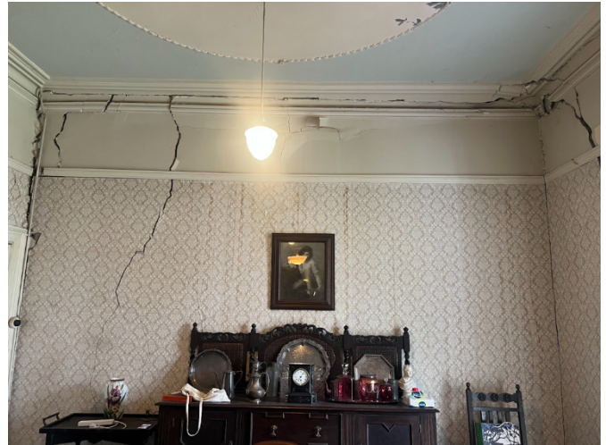
2026. Cracking to walls in dining room.
