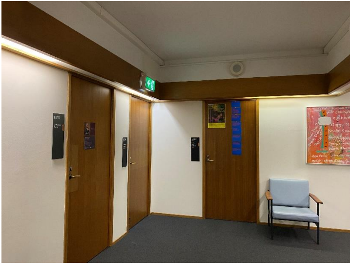
2026, Original strip lighting, encased in timber boxes & doors survive in many hallways. Source: Heritage Victoria.
