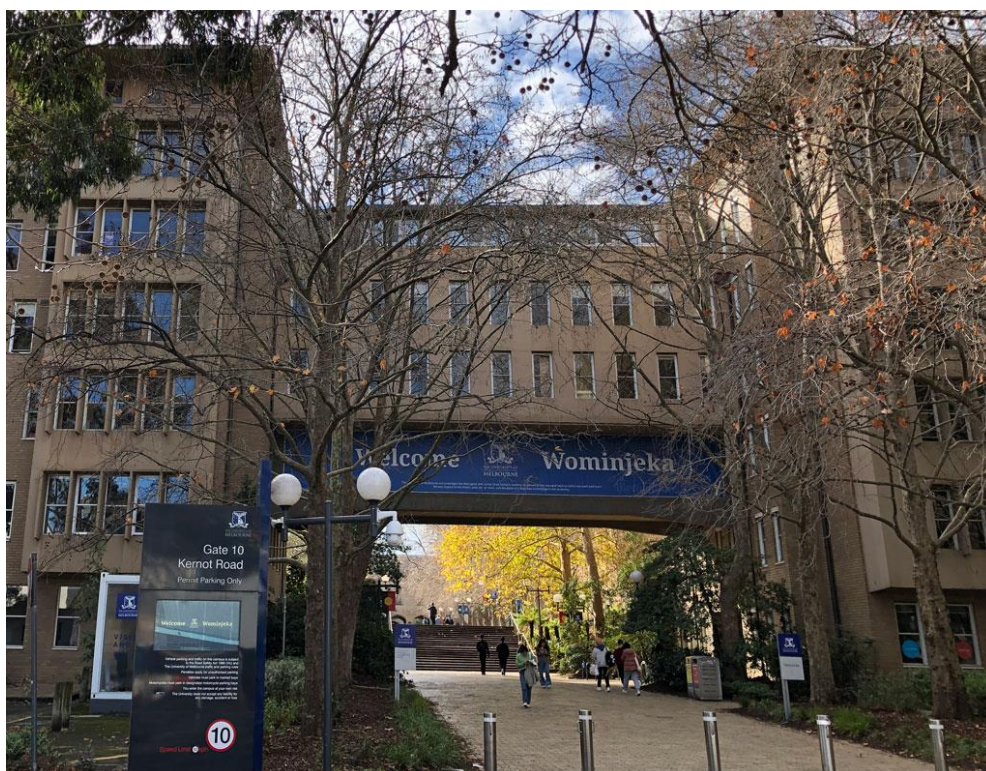
2026, John Medley Building southern elevation. Source: Fait accompli? | Butterpaper .
