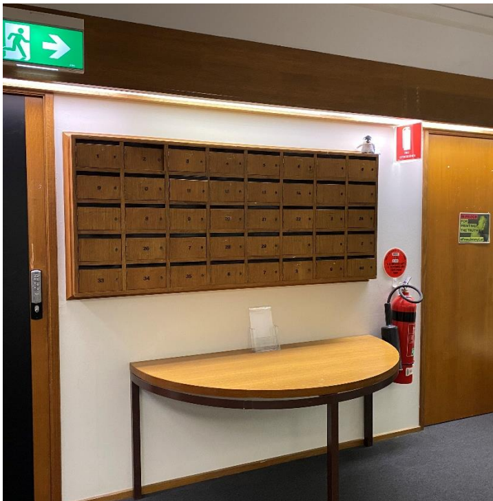
2026, Original fixtures including pigeonholes retained. Source: Heritage Victoria.
