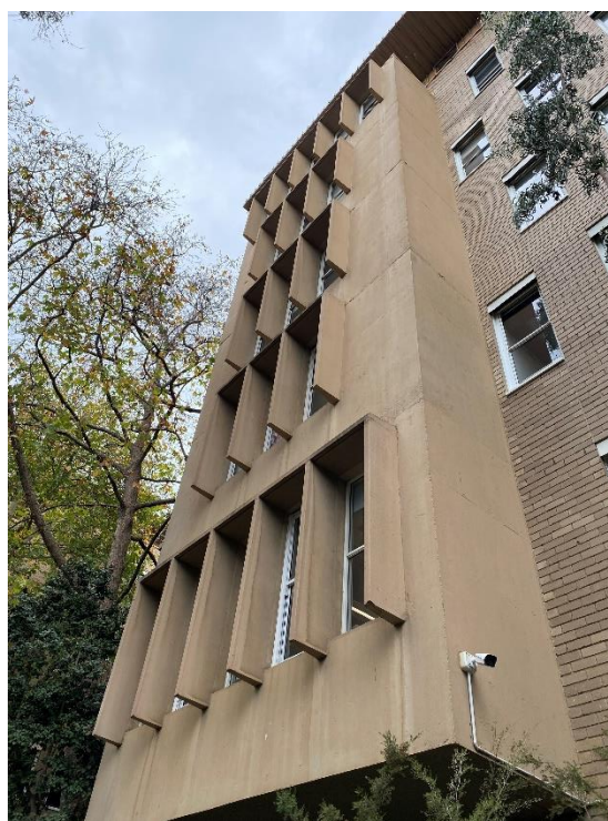
2026, Concrete cantilevered bays on west tower, with precast concrete window hoods. Source: Heritage Victoria.
