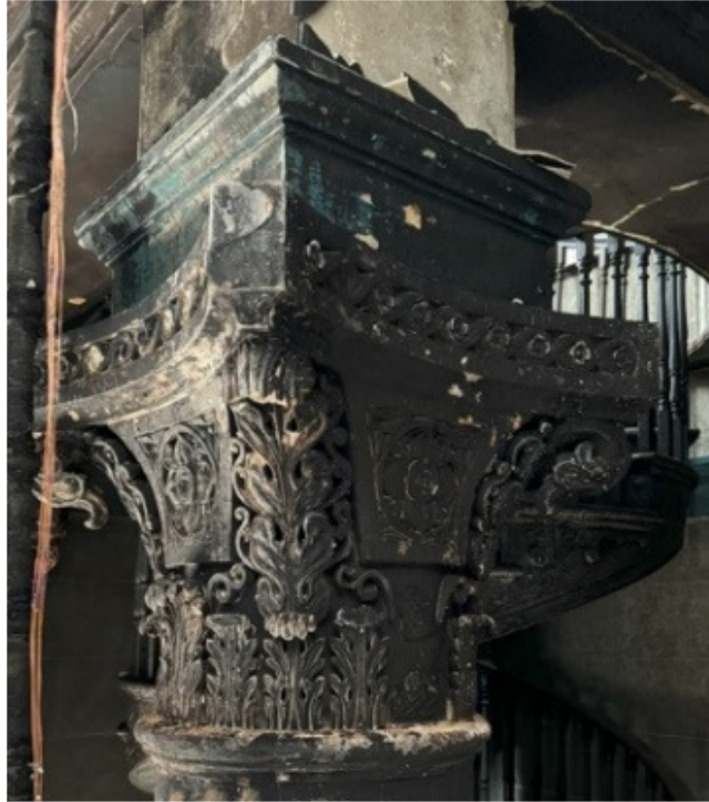
February 2024, Guan Di Hall column detail, after the fire. Source: Sophie Couchman
