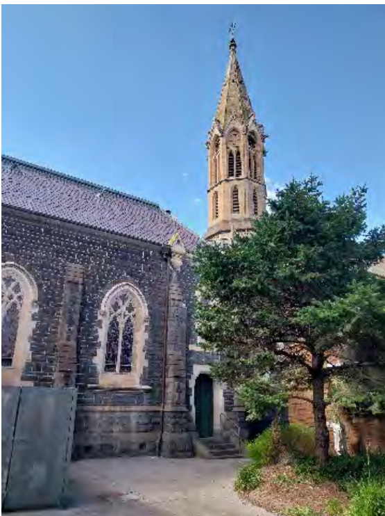
2024, View to the Convent Chapel from the aged care centre courtyard. Source: Heritage Victoria
