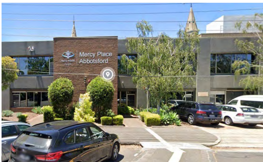
December 2020, Former Mercy Health aged care centre from Clarke Street. Source: Google streetview
