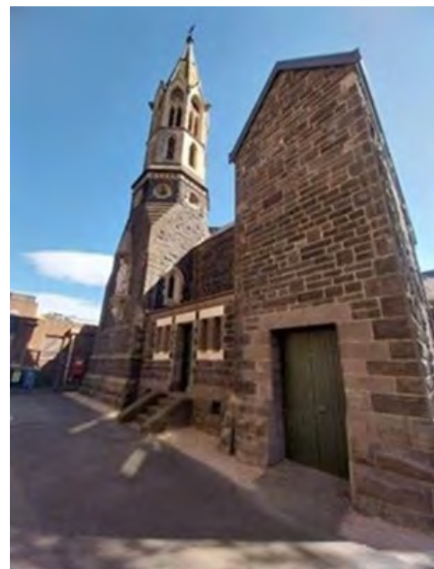
2024, South elevation of Convent Chapel. Source: Heritage Victoria
