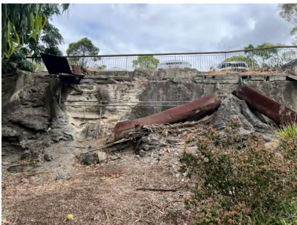
2024. Extant chutes to the western retaining wall of Bottom Factory (5).
