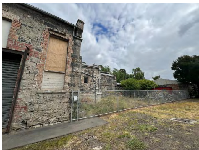
2024. Fenced off area between Building 2 (left) and Building 1 (right).
