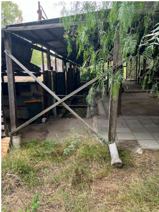
2024. Top Factory (6) middle section where pipes were loaded into steam chambers
