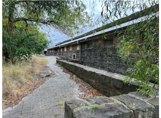
2024. Western elevation of Building 2.
