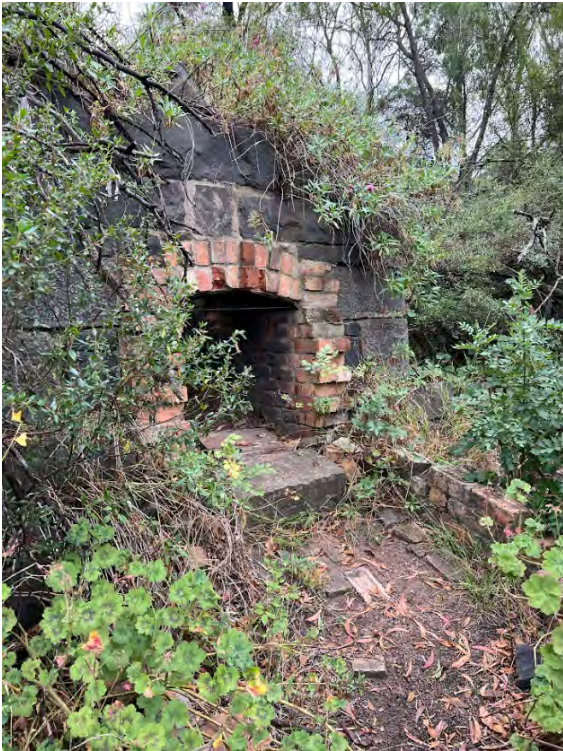
2024. Remains of chimney stack (4) between Building 2 and Building 3.
