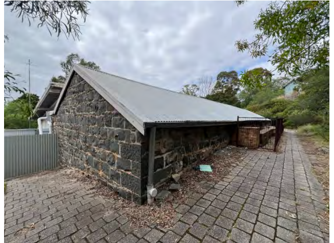
2024. Northern and western elevations of Building 3.
