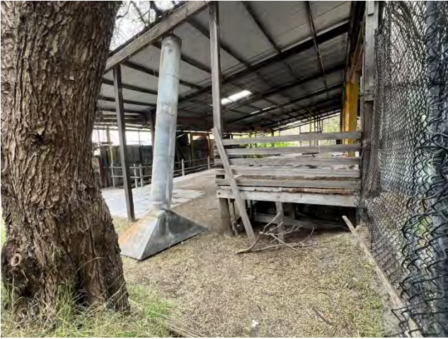
2024. Top Factory (6) timber platform.
