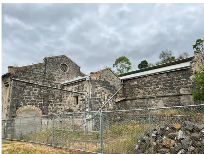
2024. Northern elevation of Building 2.
