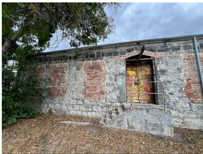
2024. Eastern façade of Building 1.
