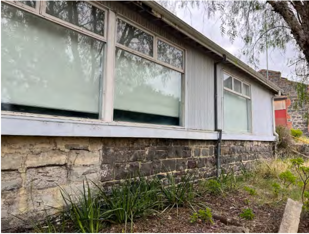
2024. Non-bluestone addition to Building 3.
