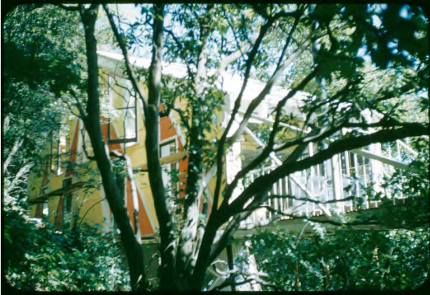
c1954, River House photographed by Peter Wille. Source: State Library of Victoria
