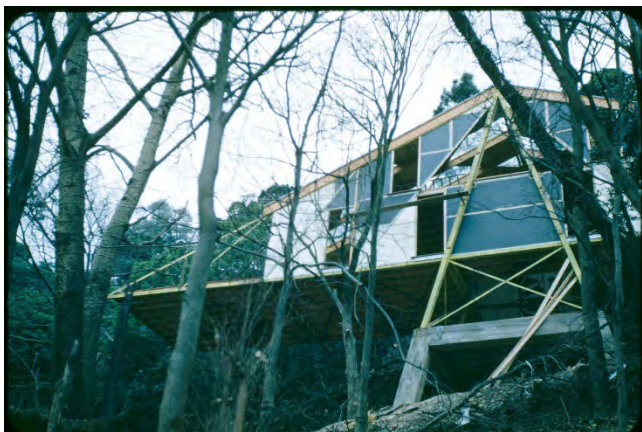
c1954, River House under construction as photographed by Peter Wille.
