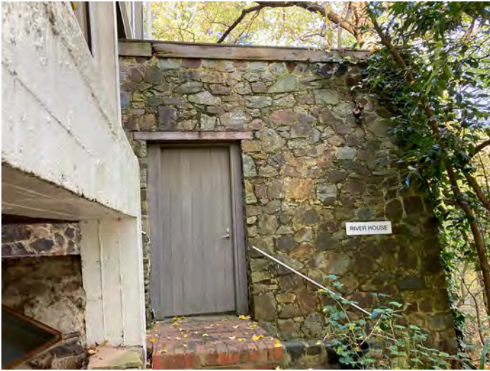
Entrance to ground level addition, c 1960s and altered 1980s.
