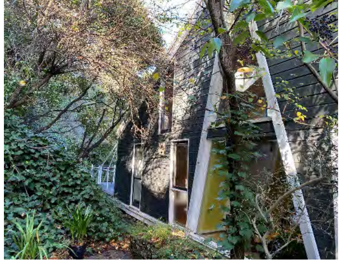
Rear, or north-east elevation of the residence.
