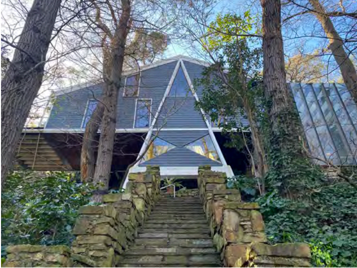
South-west elevation of residence, which faces the river.
