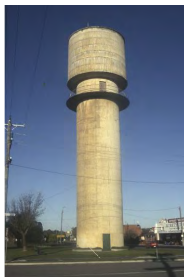
2005. Concrete water tower (1926), Bairnsdale Pumping Station. Source: Heritage Victoria
