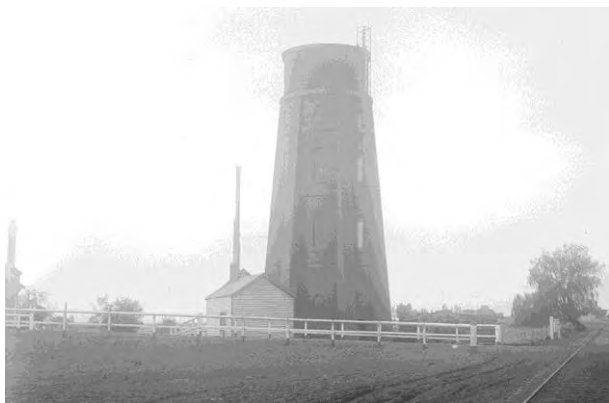
Early 1900s. The water tower as viewed from the railway. Source: Item AF00243980, New South Wales State Archives
