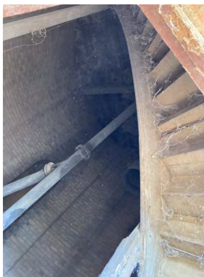
2023. Internal view of the tower.
