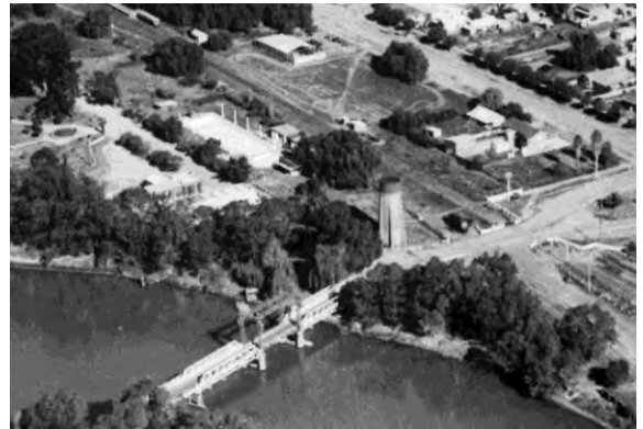
C 1920s-50s. Aerial view shows the water tower. The boiler works, boiler and engine houses adjacent to the tower and the connecting engine house and inlet pipe are removed. Source: Item rg009333, Rose Stereography Series, State Library Victoria
