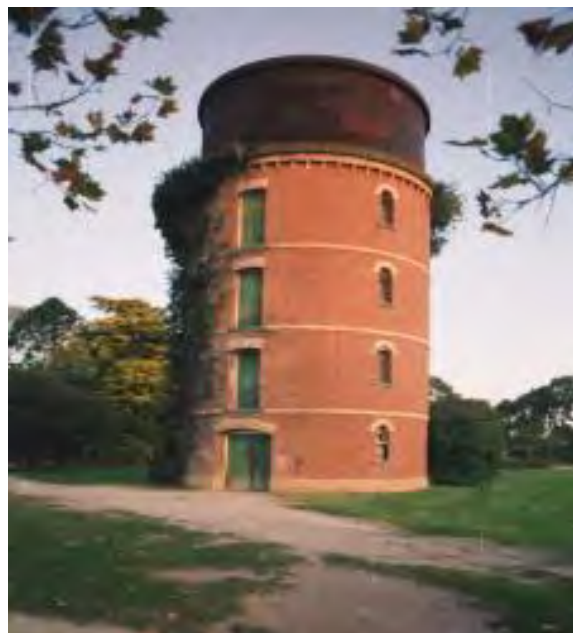
1994 Sale Water Tower, Victoria Park, Sale. Source: https://www.wellington.vic.gov.au/development/heritage-overlay-citations
