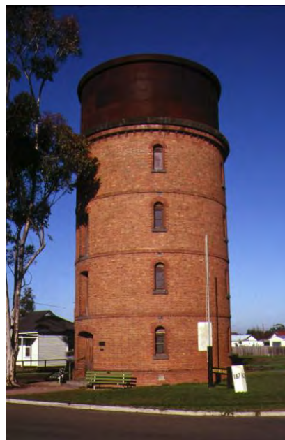
c2008. Murtoa Water Tower. Source: Heritage Victoria
