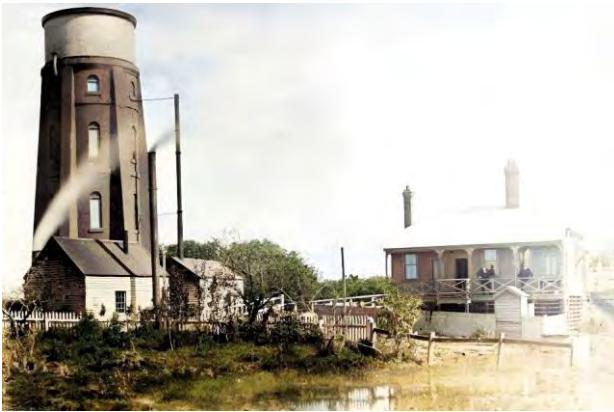
Early 1900s. Image showing the water tower from south. Note the boiler and engine houses adjacent to the tower and the connecting pipe. Source: Nominator's collection
