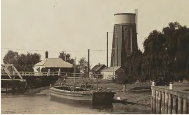
C1908. View of the water tower from north, Source: Item No 1679054, State Library Victoria
