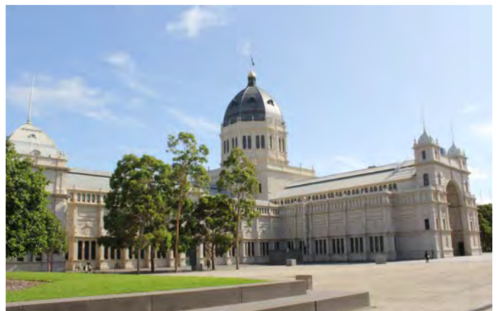
Example of a Direct View
