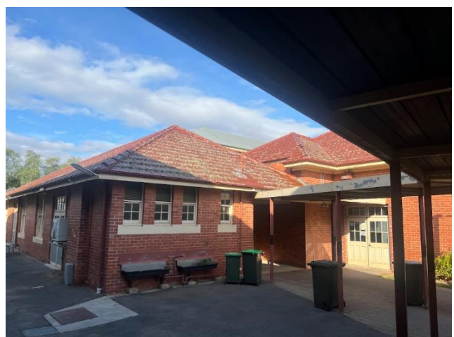
2024. Brick extension around the original sandstone building. Roof of the sandstone building visible behind tile roofs.
