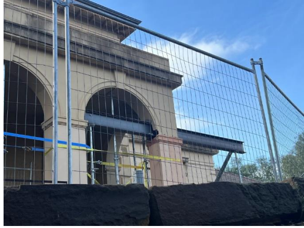
2024. Ongoing works to address subsidence.
