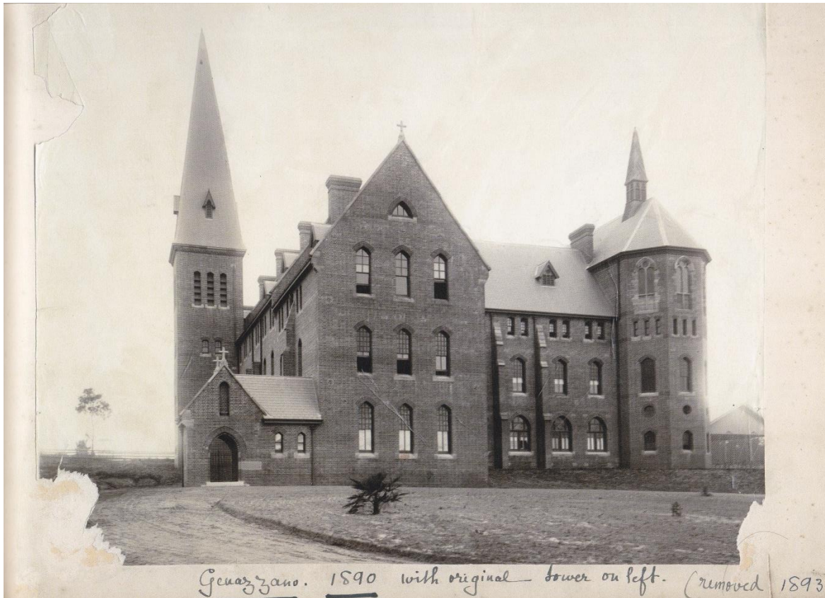
c.1891-93: Wardell Building from the northwest, prior to demolition of the spire in 1893 when it was found to be unstable. Source: Ursula M de Jong, William Wardell and Genazzano FCJ College
