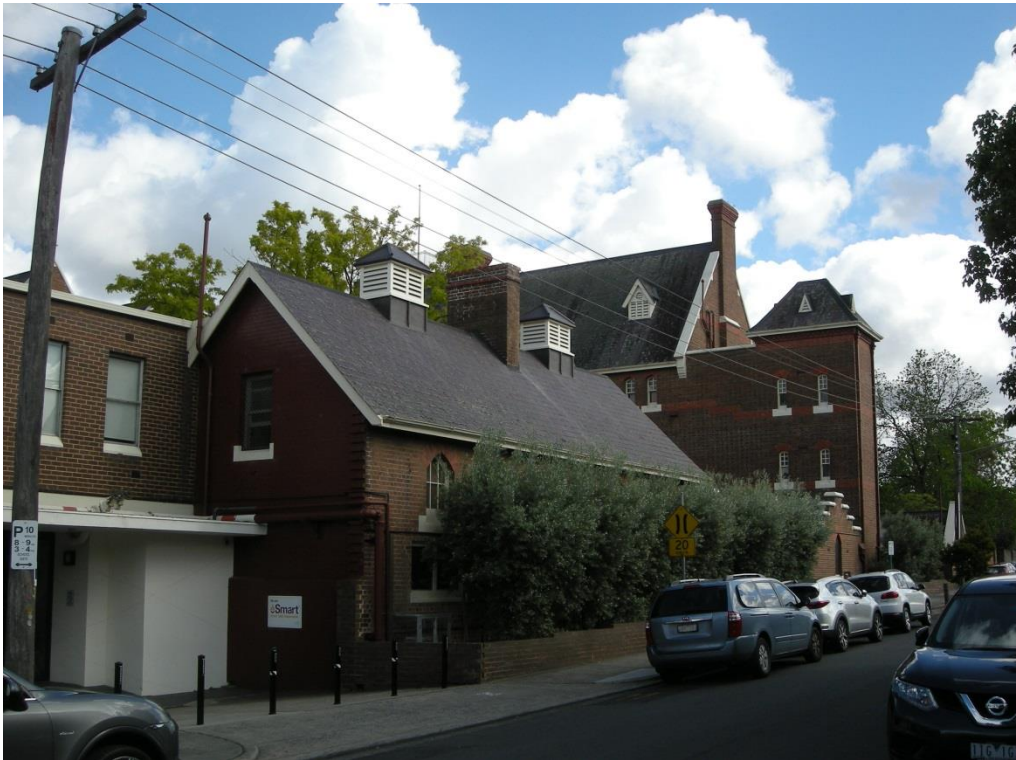
Looking northwestwards from Mont Victor Rd along the Wardell Building's east wing. Its southern end (at image's left) adjoins a two-storey portion of a 1970s building which now contains the College's public entrance. (Oct 2017)
