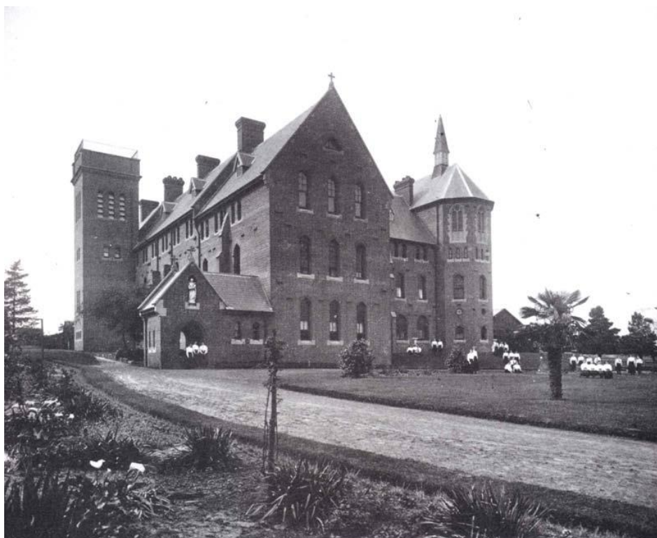
c.1910: Wardell Building from the northwest – similar viewpoint to the image on page 14. Source: And the Spirit Lingers... Genazzano – One Hundred Years 1889-1999 (via CMP, Allom Lovell & Associates)
