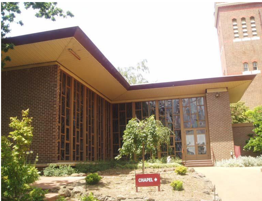
Looking from the west at the 1974 chapel. Designed by the architect Joseph McCarthy, it is a single-storey brick building with a flat roof and wide eaves.
