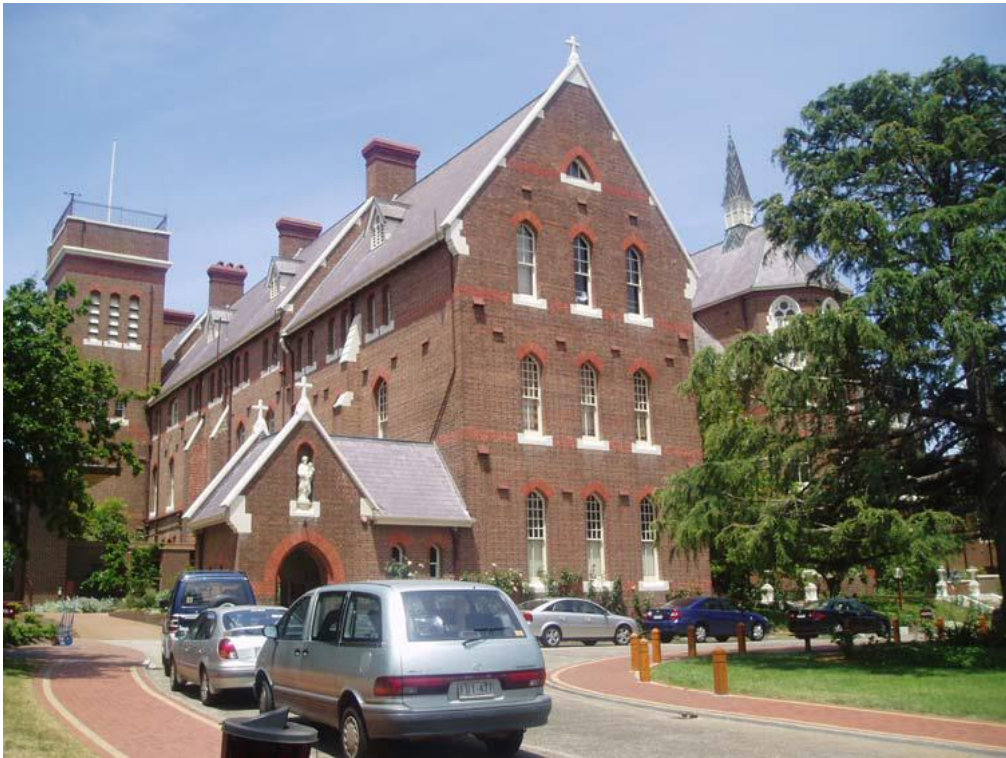
Wardell Building from northwest, with the Convent's single-storey original entrance gatehouse in the foreground. On the left is the square-plan stair tower, originally topped by a steep spire.
