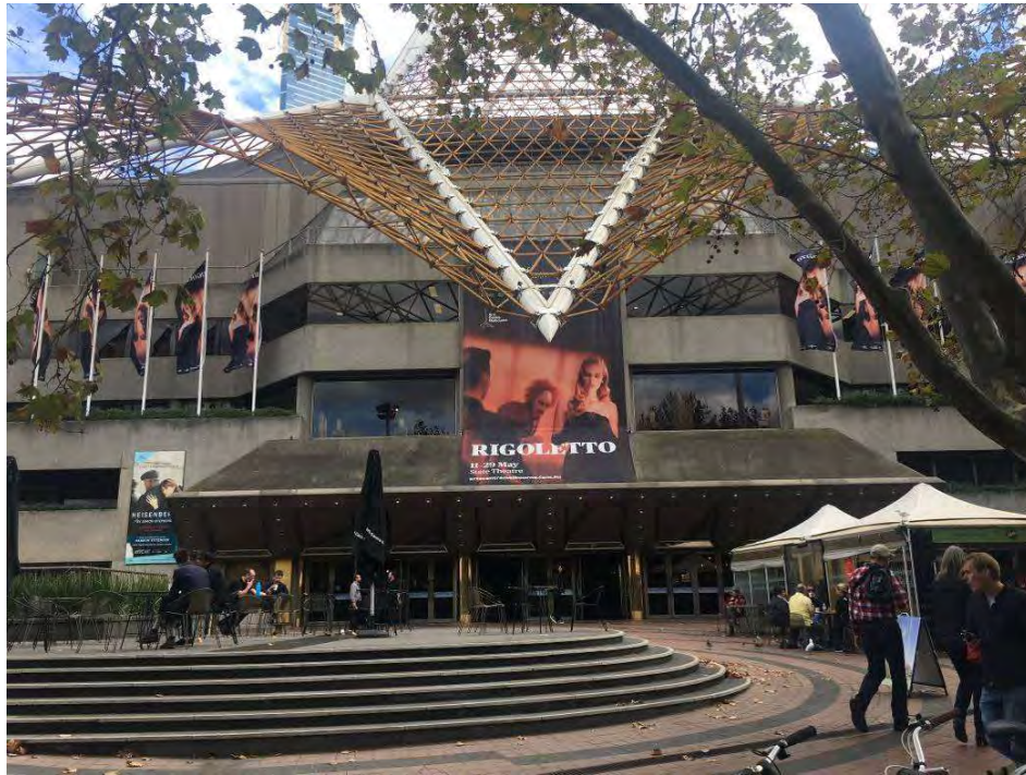
2019, Theatres Building entrance (level six) with raised 'plinth' in foreground.
