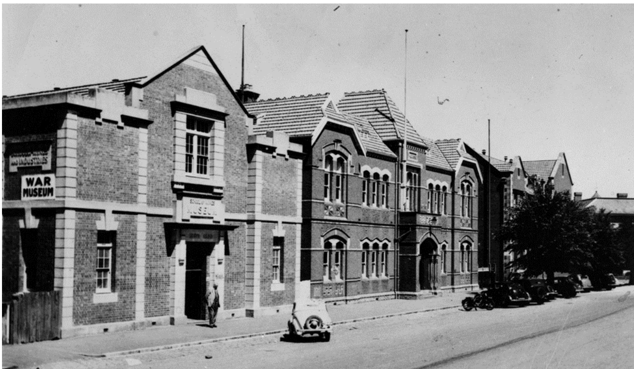
c. 1950s, School of Mines Source: Public Records Office of Victoria
