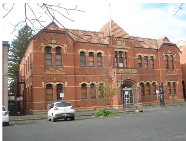
Building A, Administration Building.
