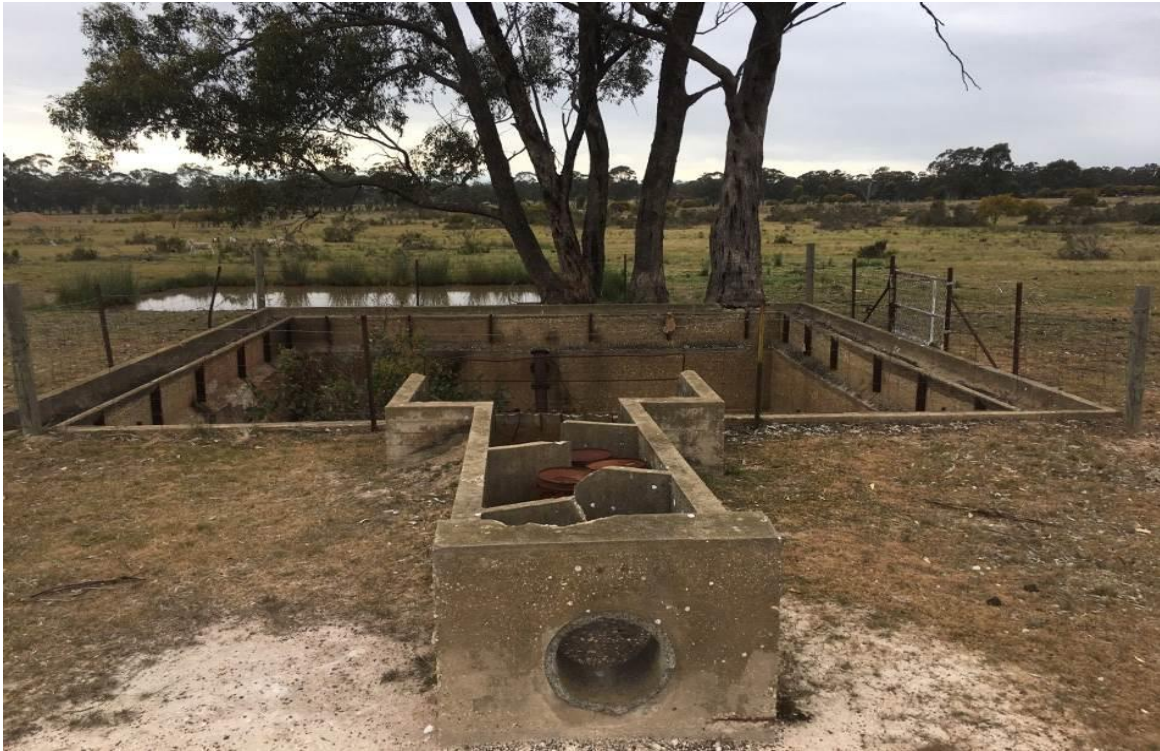
Water treatment plant, F.4
