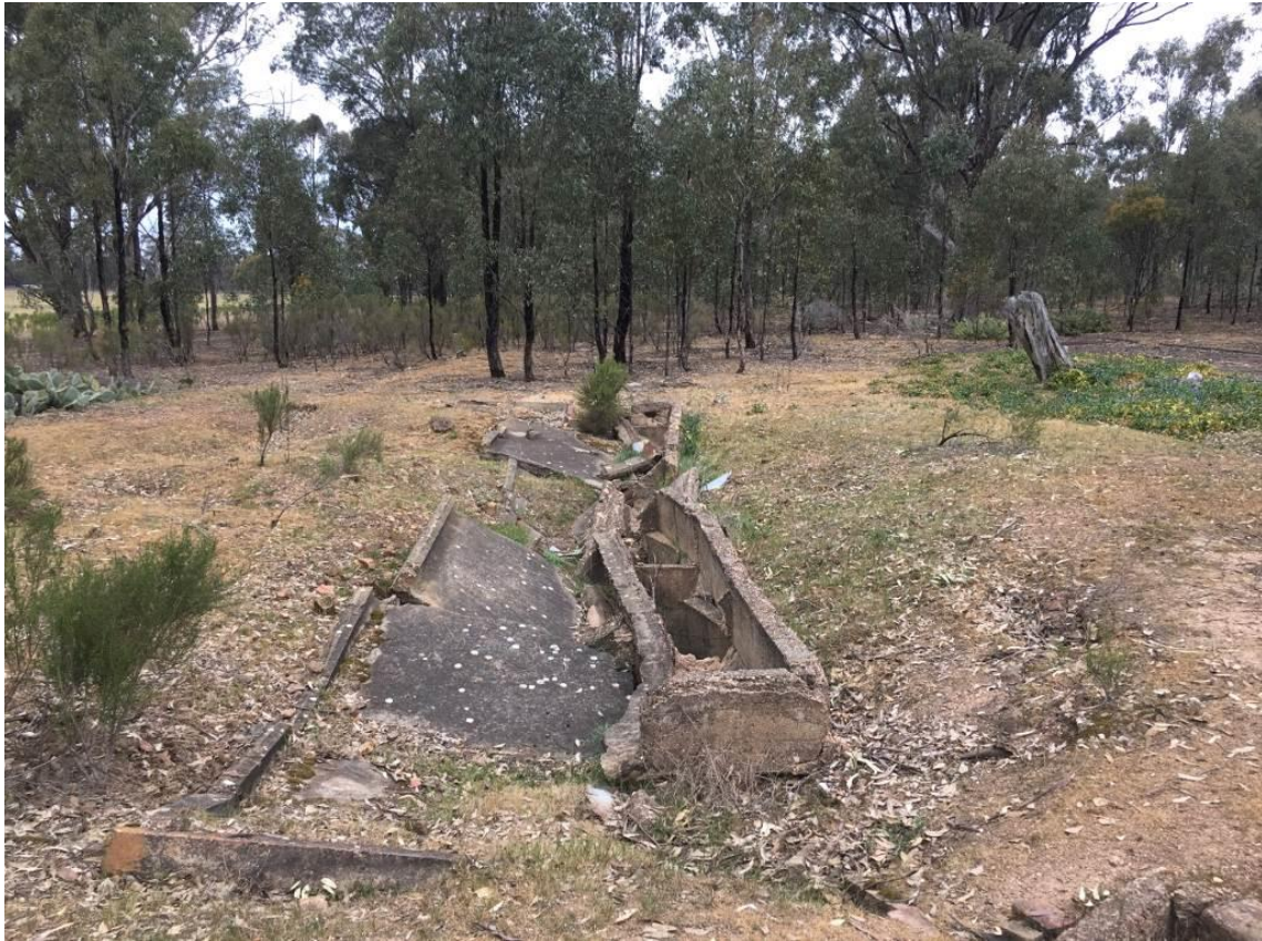
Collapsed latrine pits, F.8 (2017)
