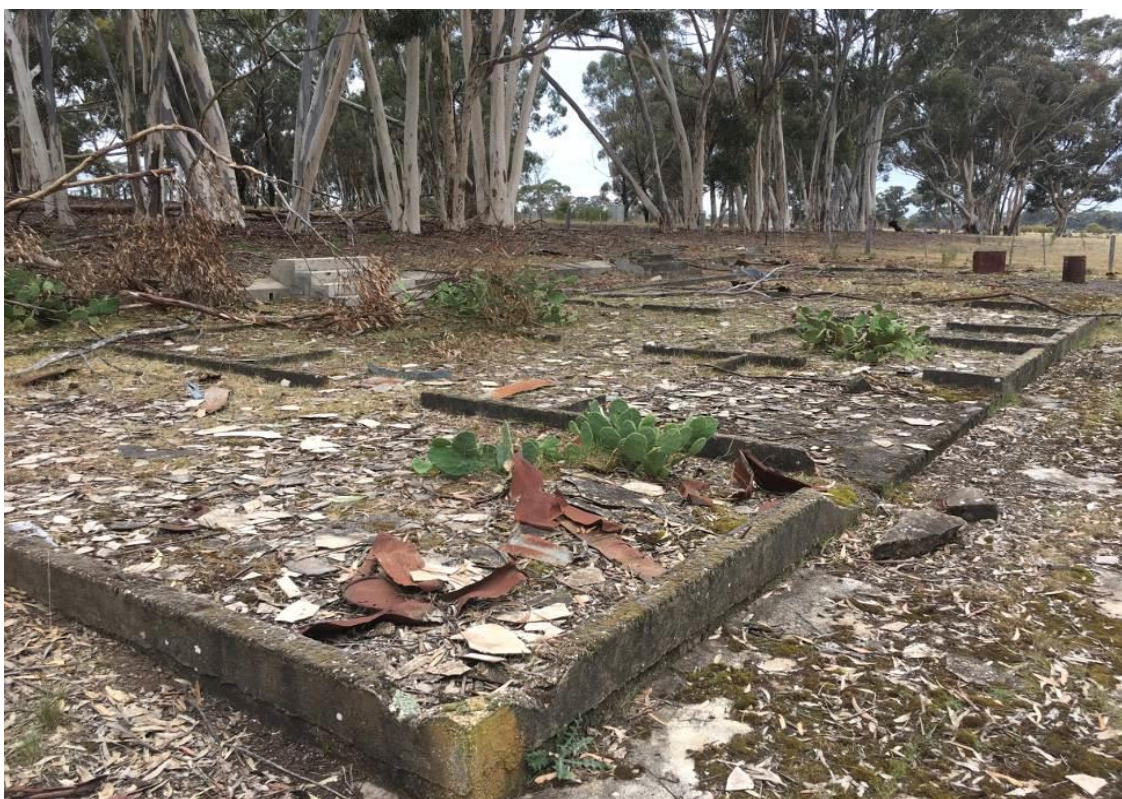
Concrete floor slabs, F8 (2017)
