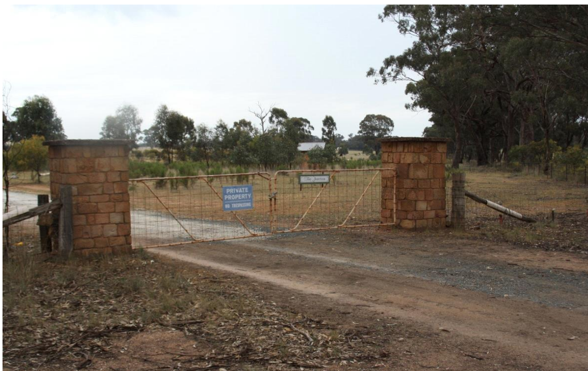
Gateway piers, F.1 (2017)
