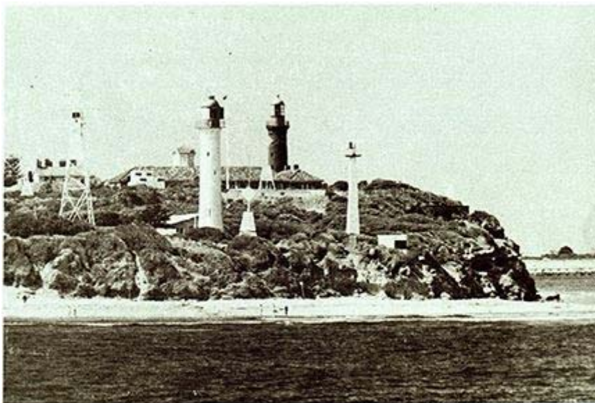
The comprehensive system of leading lights on Shortlands Bluff, Queenscliff, covering the entrance to Port Phillip Bay, is seen in this picture. The white Low lighthouse in line with the bluestone High lighthouse leads through the middle of the channel.
