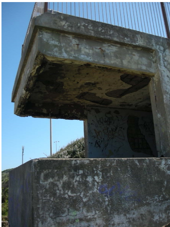
2018, World War II bunker on southern boundary.
