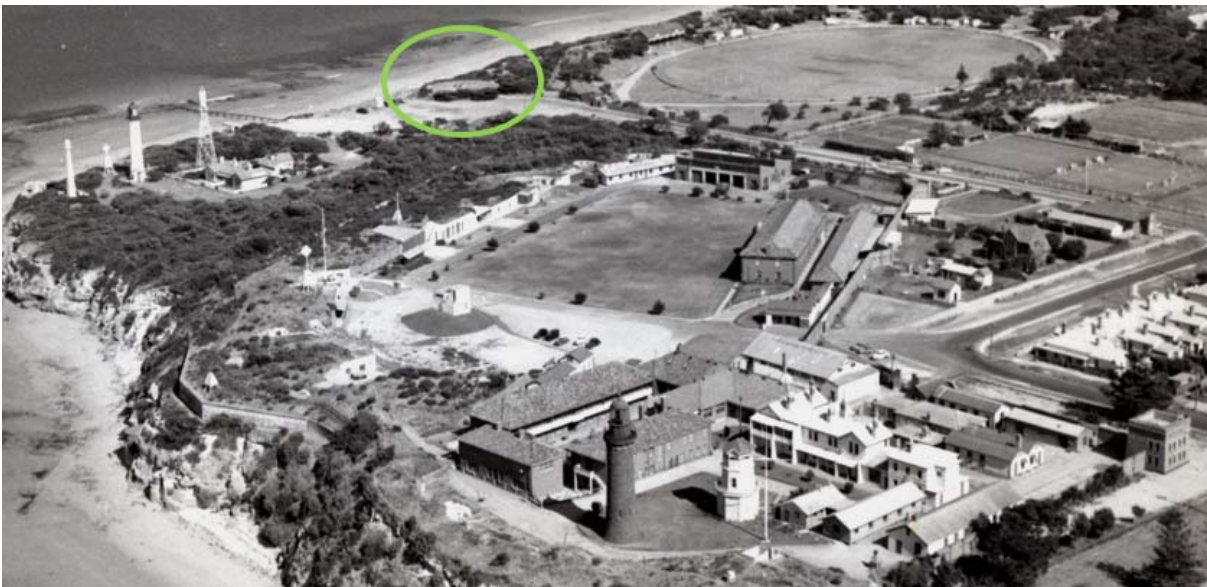
1940s, Obelisk, White Lighthouse, and towers at left; Fort Queenscliff in the foreground and the Bullring circled in green. Source: Airspy Collection, State Library of Victoria
