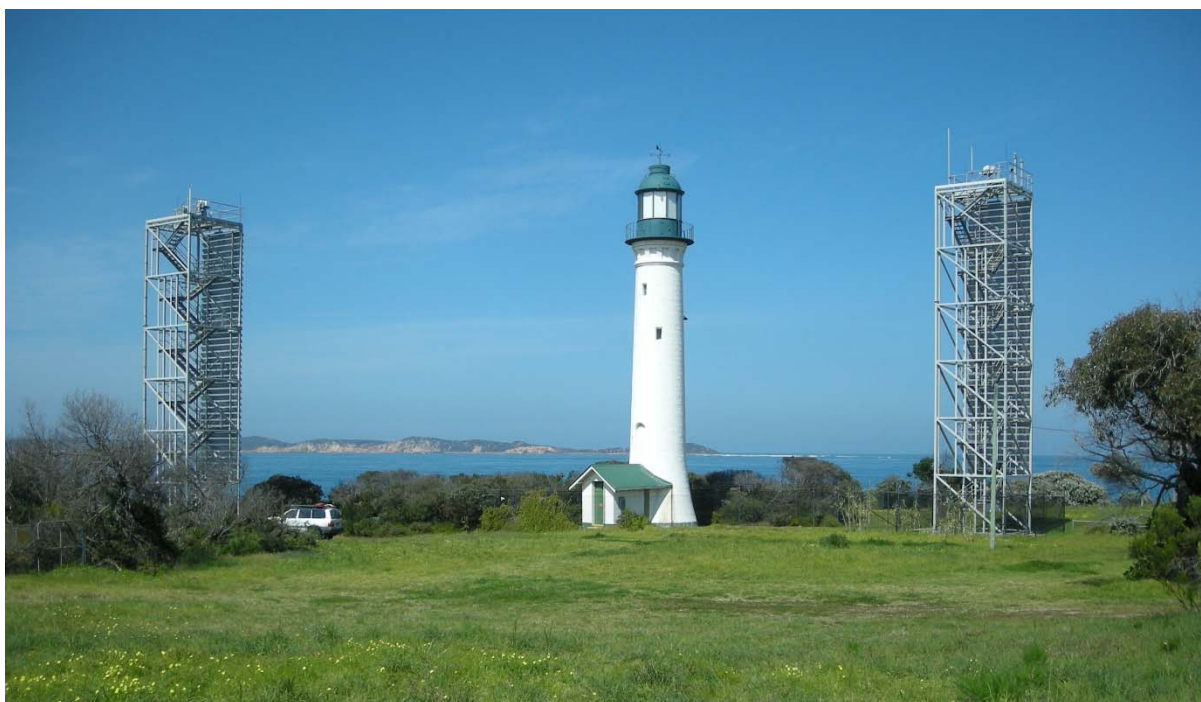
2018, Looking south-east towards Point Nepean. The White Lighthouse is in the centre. The Murray Tower is on the left and the Hume Tower is on the right. Both are replacements of earlier towers.
