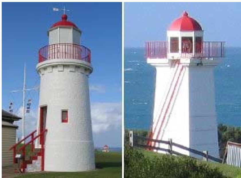
The Lady Bay Lighthouse Complex, Warrnambool. Left: Upper Lighthouse, Right: Lower Lighthouse.
