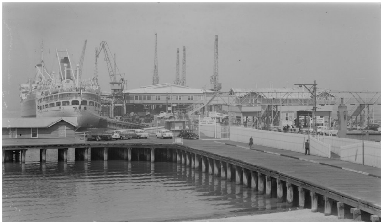
1930s, Entrance to Station Pier (Stothert & Pitt cranes in background). Source: State Library of Victoria
