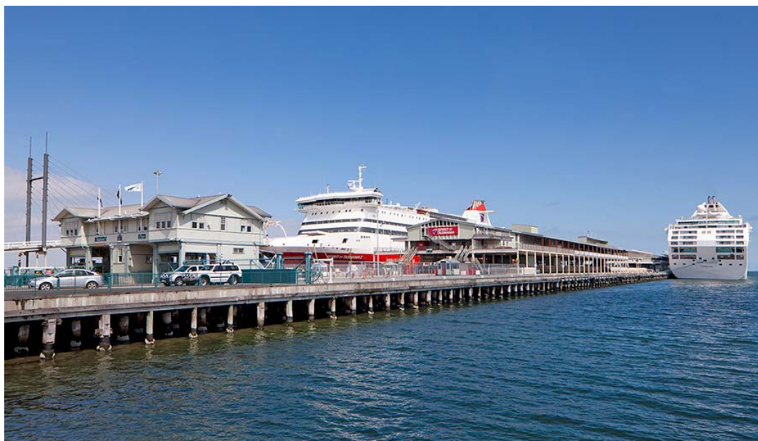
2018, Station Pier, looking south east. Source: www.lovellchen.com.au
