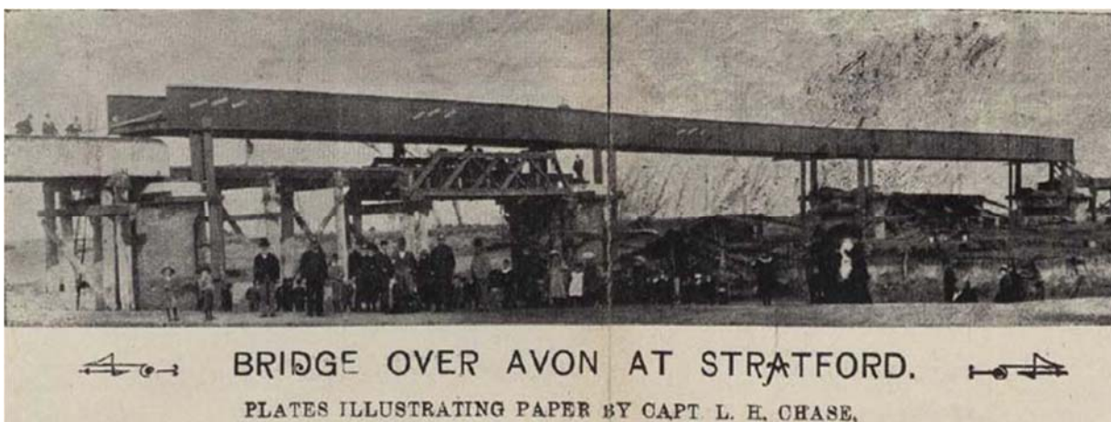
1896, The girders being lowered into place. Source: University of Melbourne
