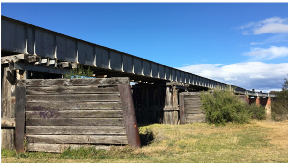
Avon River Rail Bridge (August 2018)
