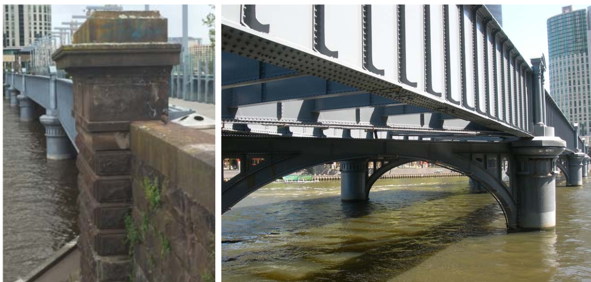
Sandridge Railway Line Bridge (VHR H0994)
