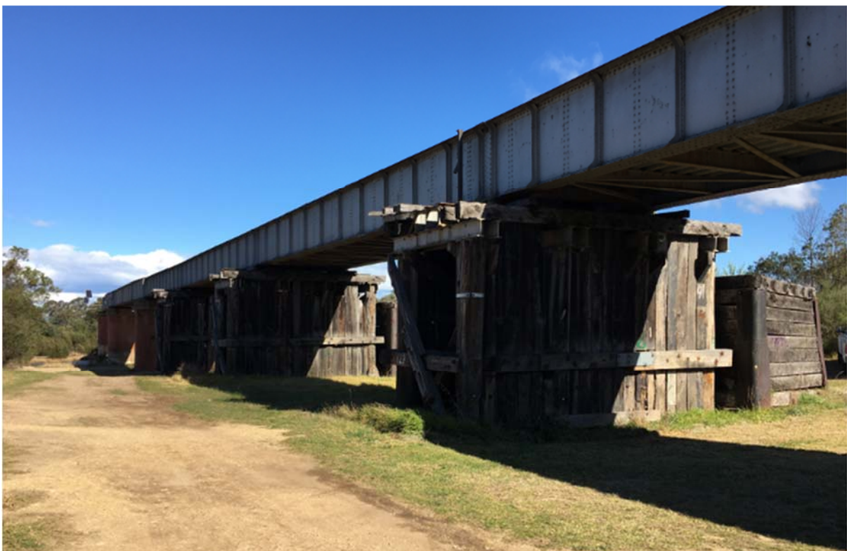
2018, Timber cutwaters and piers of the 1888 section, looking south-west.
