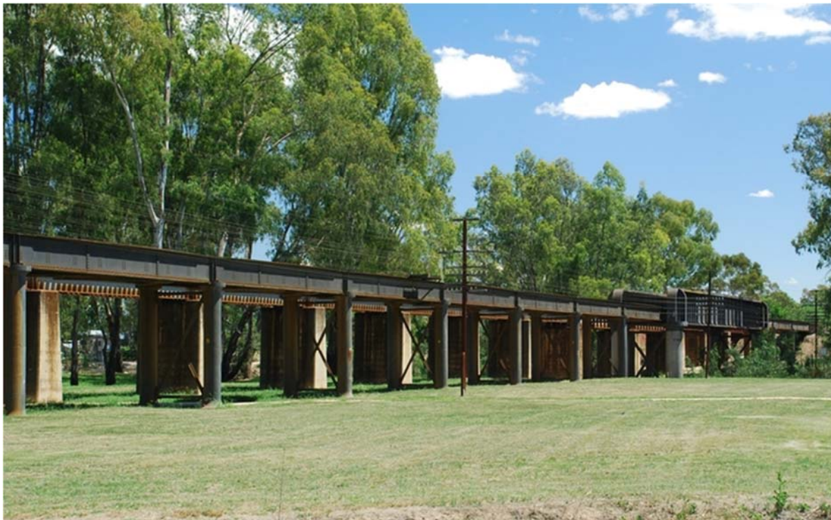
Rail Bridge, Broken River, Benalla (VHR H1061)
