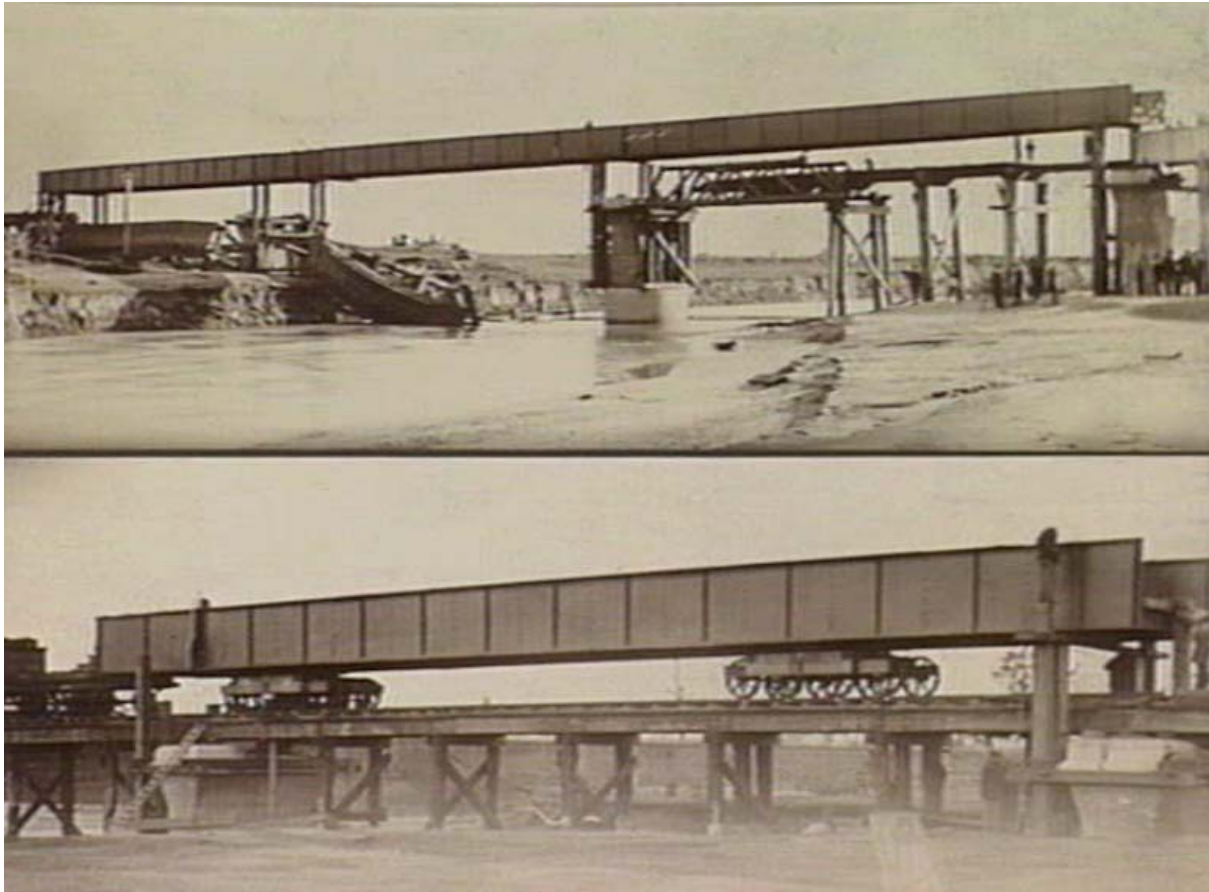
1896, Girders being moved into place with trolleys. Source: State Library of Victoria
