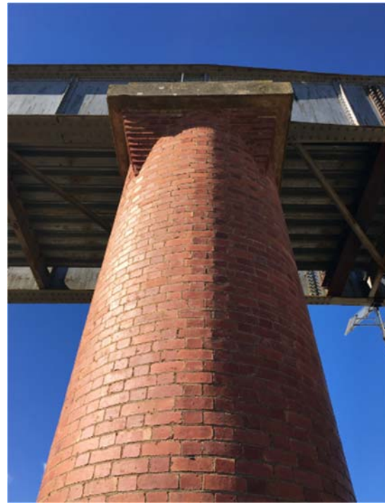
2018, Masonry pier to the 1896 section showing brick detailing to tops.
