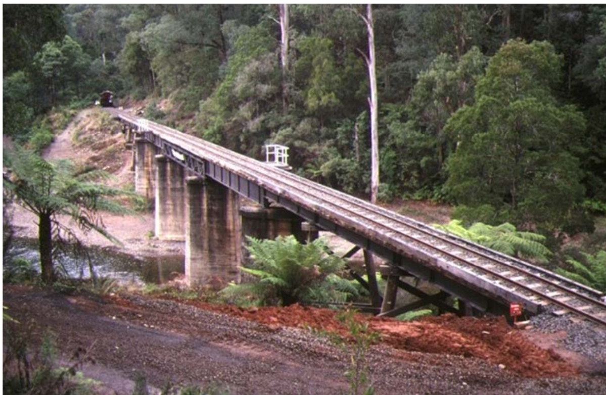
Thomson River Rail Bridge, Walhalla (VHR H1443)
