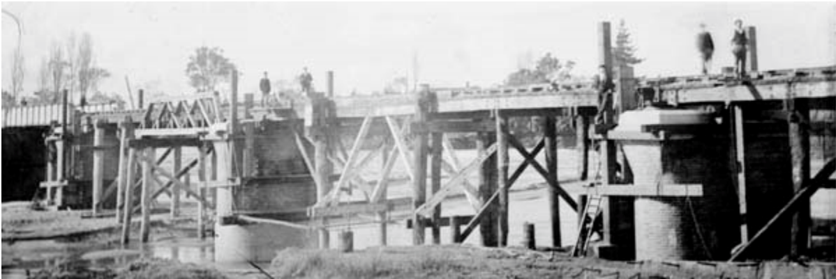
1896, Construction of the masonry piers.
