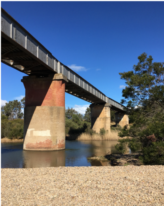
2018, The extension over the new course of The Avon River (1896 section).
