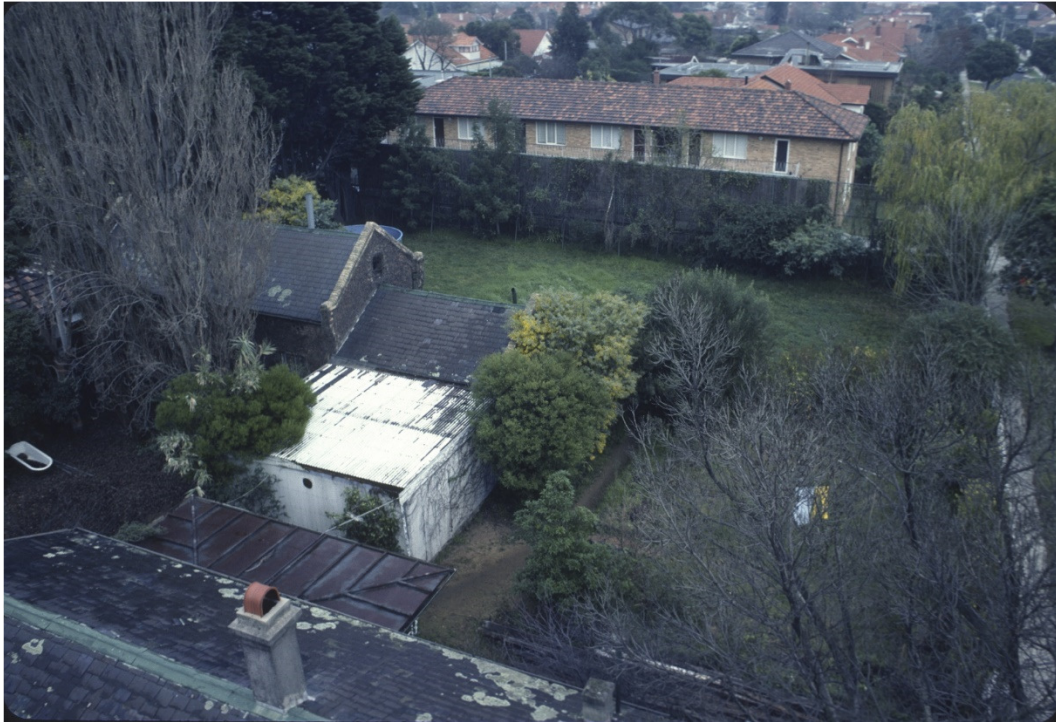
c. 1978, view from tower towards stables, which then consisted of three adjoining structures. Note that the east-west wing along Halstead Street had not been built.
