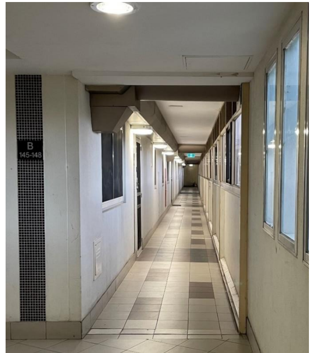
Corridor B, Level 12, 33 Alfred Street. Original balcony access to flats infilled with metal and glazing to form corridor (25 June 2025).
