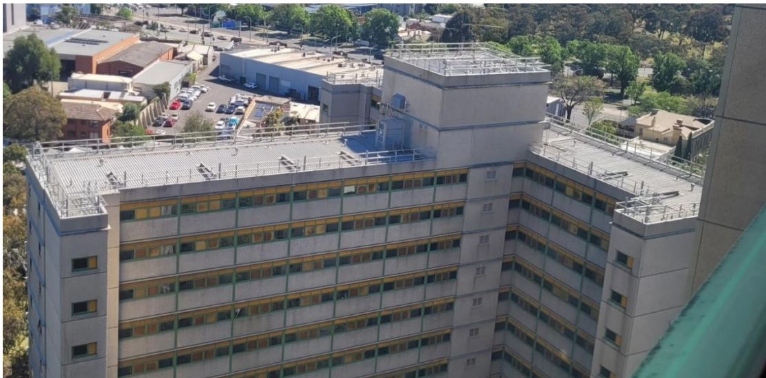
Looking onto the T-type tower from the 19 th floor of 12 Sutton Street. Note the infill of glazing and yellow metal grills that now enclose the originally open balconies (28 October 2025).
