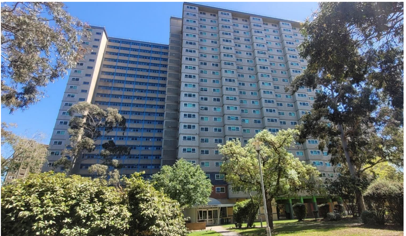
12 Sutton Street, Z-type 20-storey high-rise. Living rooms with three windows project from the façade. The infilled balconies of the rear wing can be seen on the left (28 October 2025).
