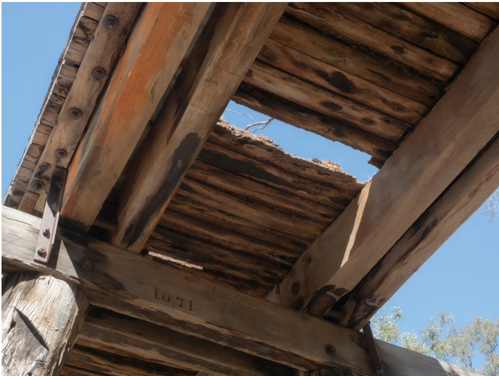
2025, view of longitudinal stringers above crossheads, Source: Explore Nelson And The Glenelg River Victoria Facebook group.
