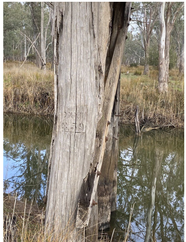
2025, bridge abutment on southern end, Source: Heritage Victoria. 2025, Markings on pile that detail replacement, Source: Heritage Victoria.
