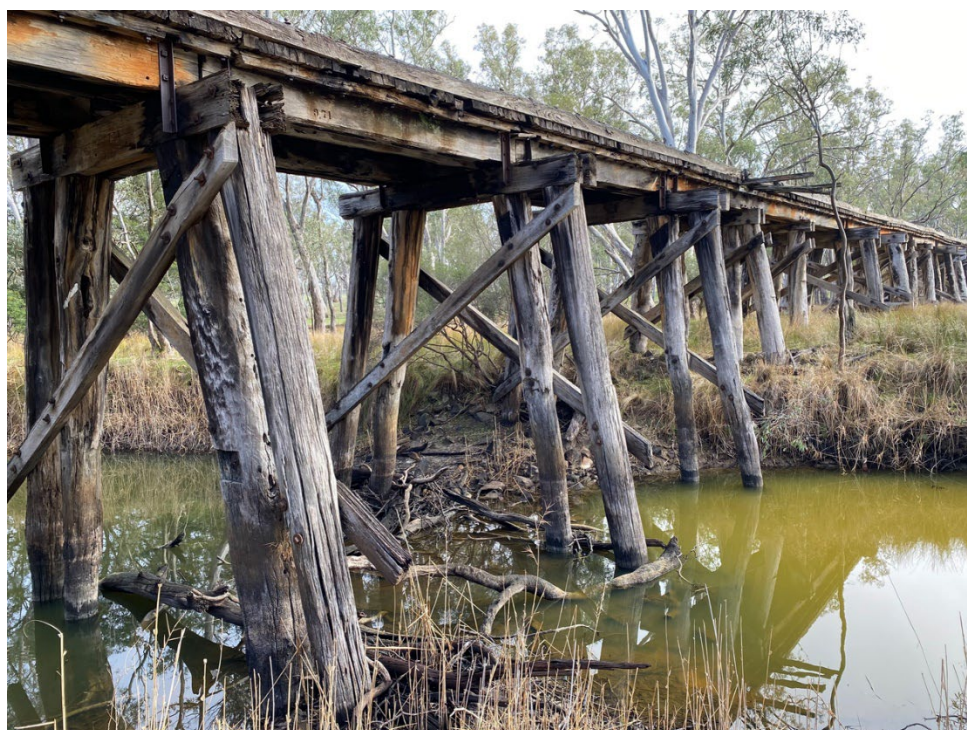
2025, close up of southern trestles. The two short horizontal beams at right near the sapling are the last remains of a deteriorated timber safety platform. Source: Heritage Victoria.
