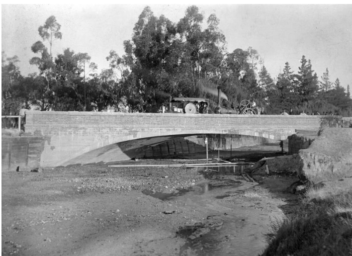
1901. First failed Kings Bridge (single, long span bridge) Test Source: University of Melbourne Archives [1964.0012] Records and photographs of the Reinforced Concrete and Monier Pipe Construction Co. Pty Ltd.
