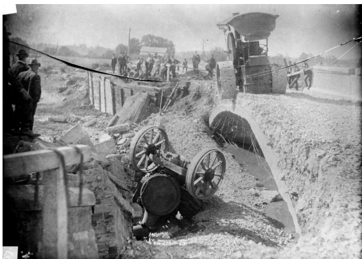
1901. Kings Bridge collapse. Source University of Melbourne Archives [1964.0012] Records and photographs of the Reinforced Concrete and Monier Pipe Construction Co. Pty Ltd.
