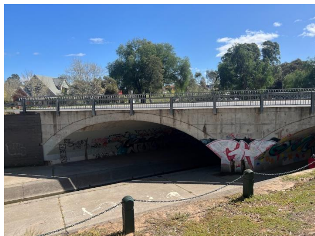
2024. 2004 section of the bridge viewed from the south.
