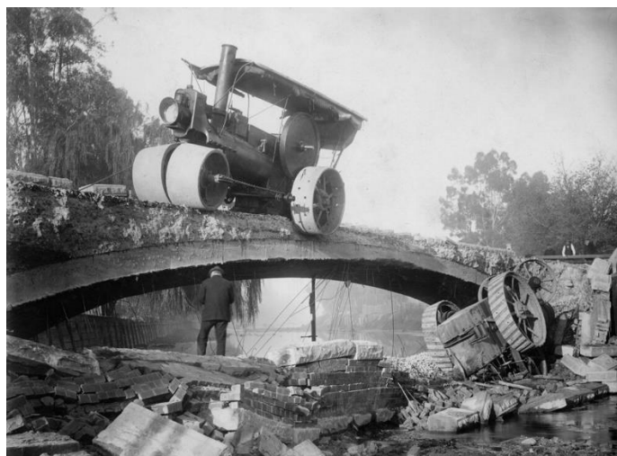
1901. First Kings Bridge collapse. Source: University of Melbourne Archives [1964.0012] Records and photographs of the Reinforced Concrete and Monier Pipe Construction Co. Pty Ltd
