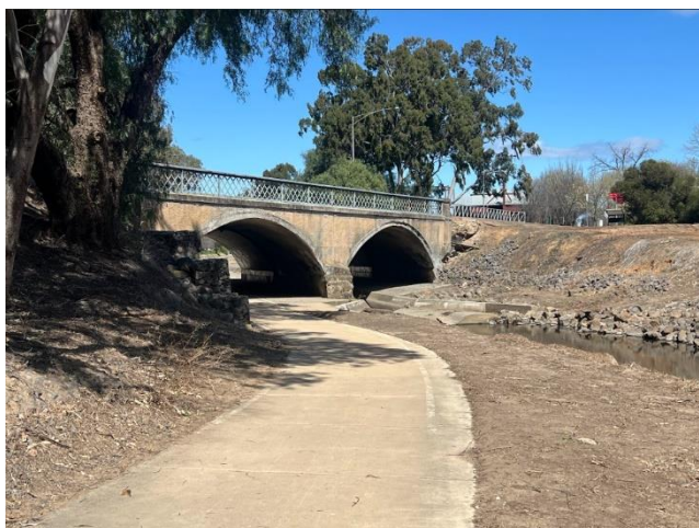
2024. 1902 section of the bridge, viewed from the north (upstream).
