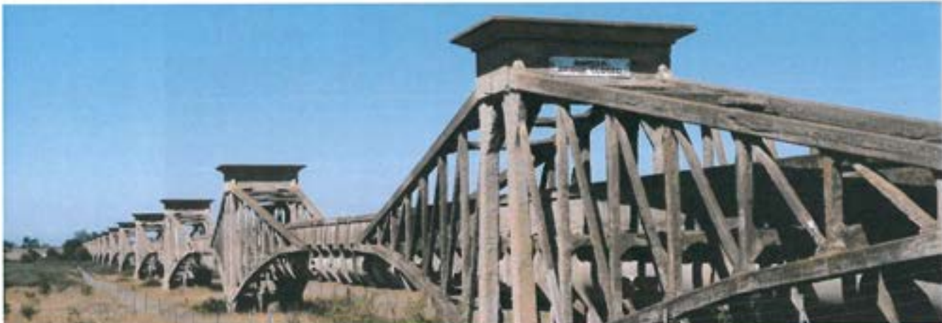
Ovoid Sewer Aqueduct
