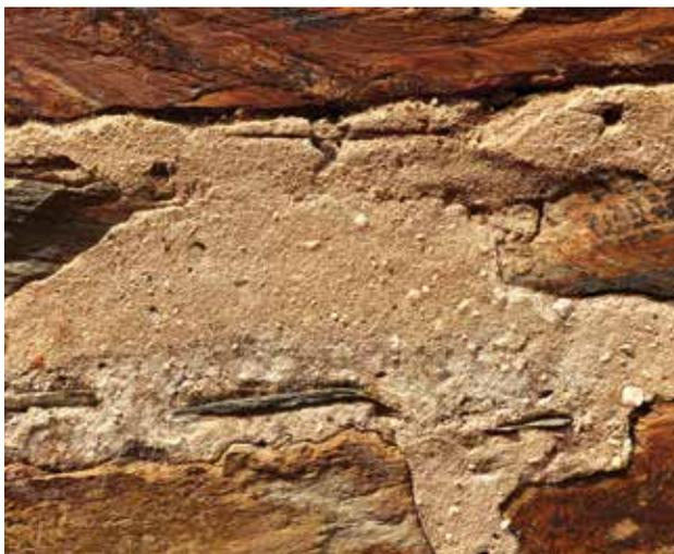
**Figure 60: Flushed up pointing.**
