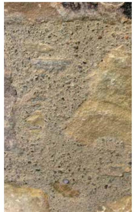
**Figure 72: Tamped joints in rubble stonework.** The tamped joints have a weathered or aged appearance with exposed sand grains. Without tamping, the colour would be that of the binder and finer sand grains. Also note the small pinning stones pushed into the mortar during repointing (see Chapter 22).
