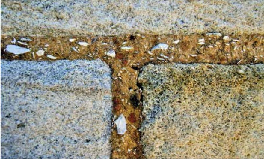
**Figure 28: Shell fragments in an 1830s mortar.** The rest of the aggregate is a very fine, silty sand with some darker gravel particles.
