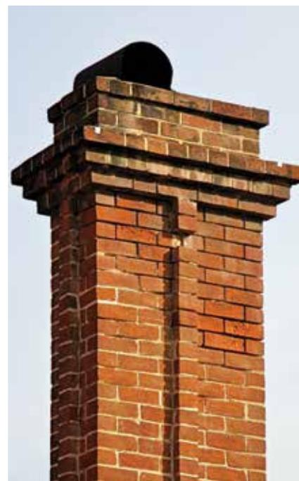
**Figure 34: Which mortar?** Because chimneys are more exposed, the initial response may be to use a stronger mortar than the original, but here the bricks are deteriorating, requiring a weaker, sacrificial mix (type 5).
