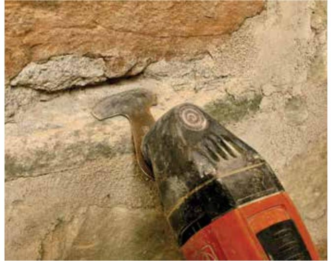
**Figure 65: Oscillating-blade tools.** These enable removal of moderately hard mortars while maintaining good control, reducing the risk of overruns. They are also much safer to use than rotating tools and produce less dust.
