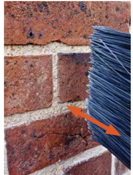
**Figure 71: Tamping the joints.** Tamping with a stiff-bristled brush (such as this churn brush) produces an aged appearance.
