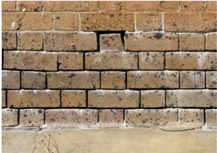
**Figure 76: Mortar loss due to dissolution.**
