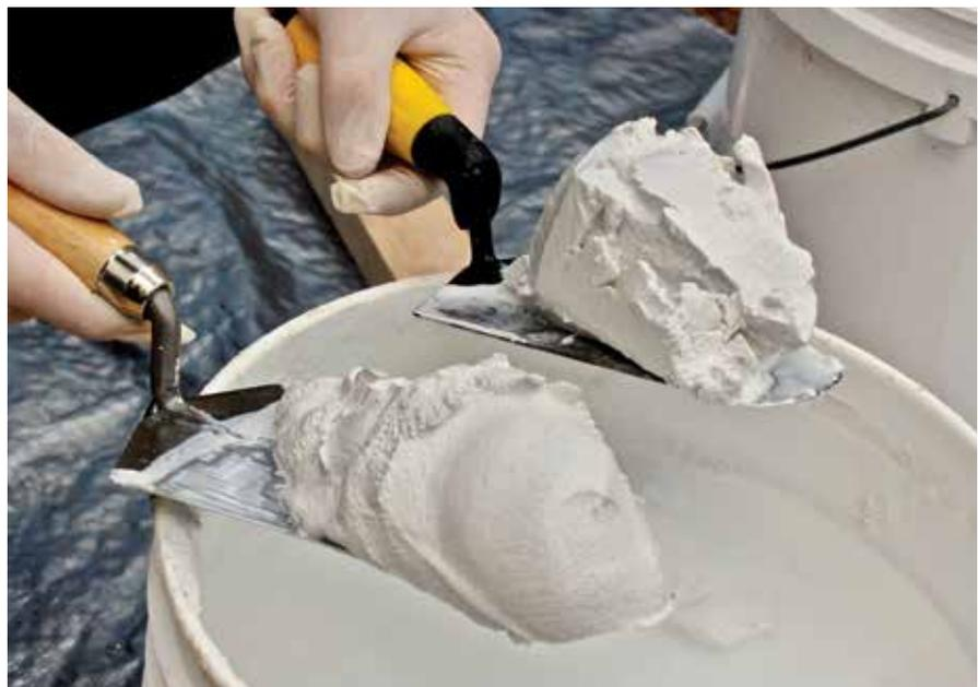
The densities of hydrated limes range from 350–640 g/L: that is, from about half to the same amount of lime per litre as in a dense putty. This has to be taken into account when batching: to make a mortar equivalent to a 1:3 mortar made with a dense putty may require a mix as rich as 1:2 hydrated lime to sand.
