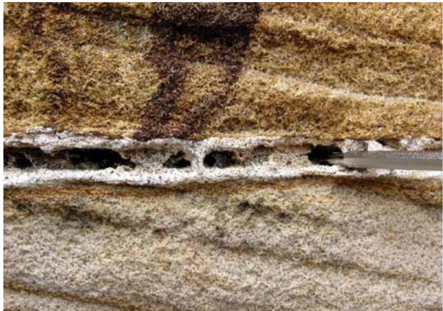
Deep joints should be filled in layers of no more than 30 mm at a time, and at least three days allowed for initial hardening of lime mortars before applying more. Pre-wet between layers and provide protection and good curing conditions (see Chapter 24 ‘Protection and curing’). Because of the slow carbonation of lime in deep joints, it may be appropriate to include a pozzolan (or use a natural hydraulic lime) in the mortar. This will depend on compatibility with the masonry units.
