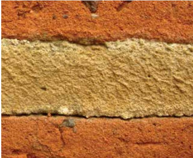
**Figure 38: Original surface of a sticky mortar.**
