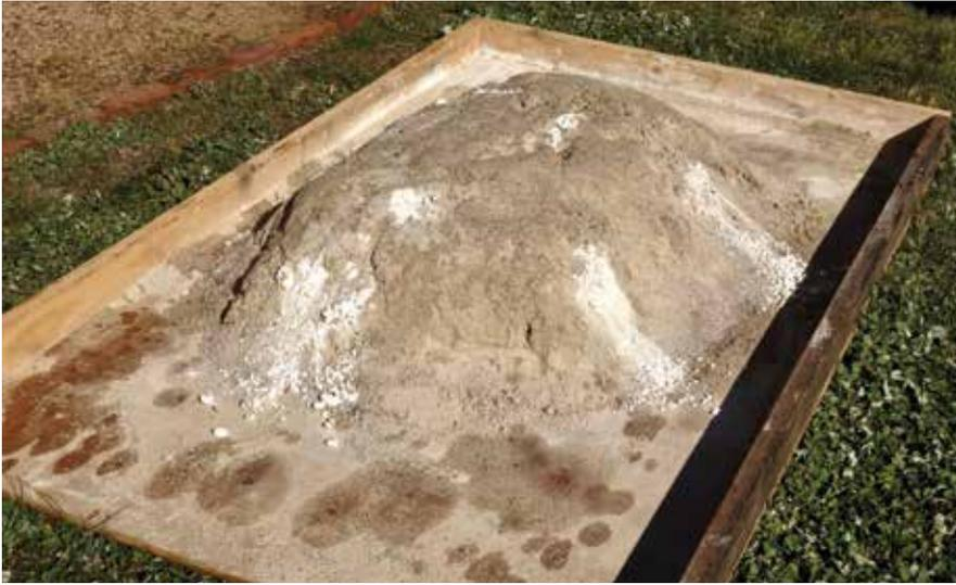
**Figure 63: Sand-slaking quicklime.**
