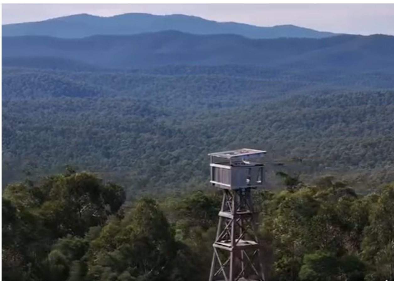
2024, drone view of Mount Little Dick Fire Tower.
