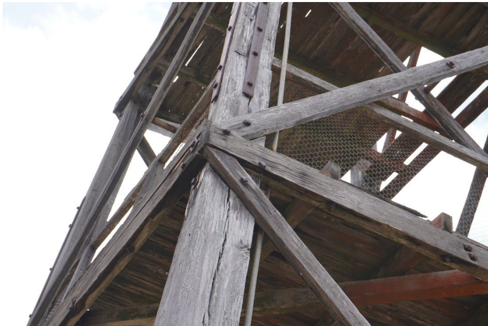
2025, detail of Mount Little Dick Fire Tower. Source: Andrew Martin, DEECA
