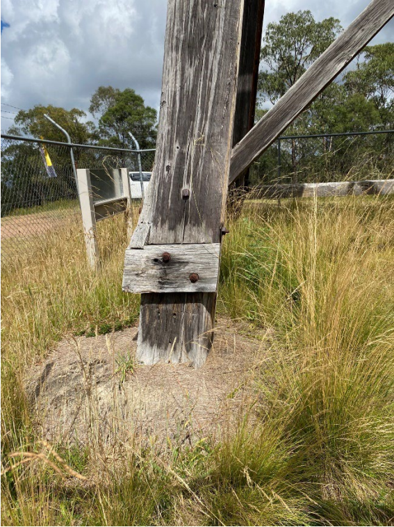
2025, the base of Mount Little Dick Fire Tower. Note that the main horizontal member has been removed on this side. Source: Heritage Victoria
