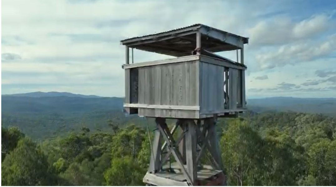
2024, drone view of Mount Little Dick Fire Tower.
