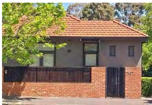
2024, Dormitory (Building 2), Cardigan Street. Source: HV
