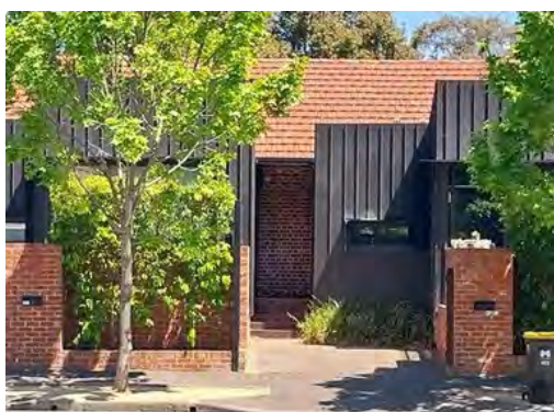
2024, Dormitory (Building 3), Cardigan Street. Source: HV
