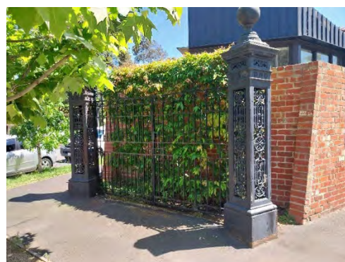
2024, wrought iron gates (1940) cast iron gateposts (origin unknown). Behind is the modern extension to the Baby Health Centre (Building 4). Source: Heritage Victoria
