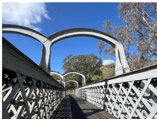
2024. Wrought iron arches, 1997 extension of height visible.
