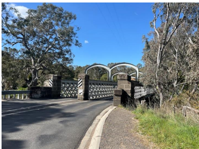
2024. Redesdale Bridge from the western approach.
