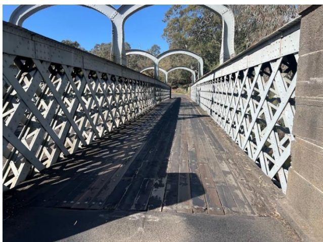
2024. Timber decking to bridge roadway.
