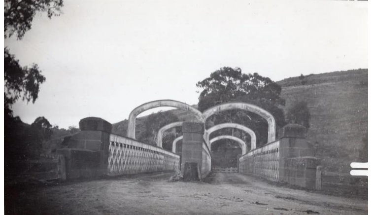
1914. Redesdale Bridge (prior to arches being raised in 1997). Source: VicRoads Association Country Roads Board Early Days.
