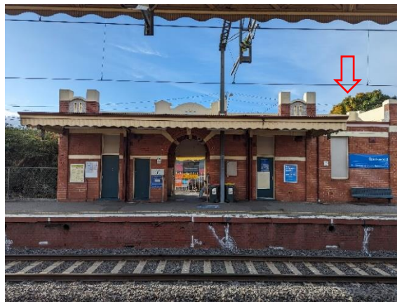
2025, platform elevation of the downside station building. The 1940s addition is indicated with an arrow. Source: GJM Heritage.
